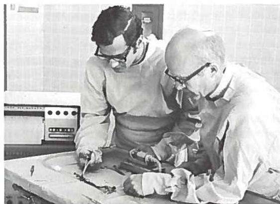
**Measuring blood pressure and flow characteristics in an excised canine aorta.**
