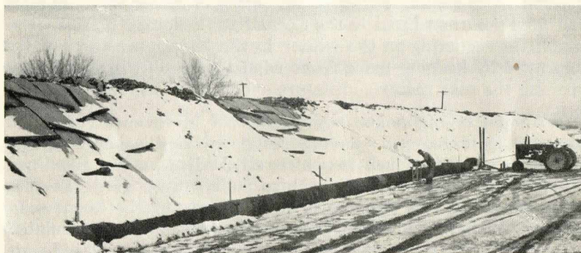
Night air blown through this experimental beet pile succeeded in lowering the temperature of the pile.
