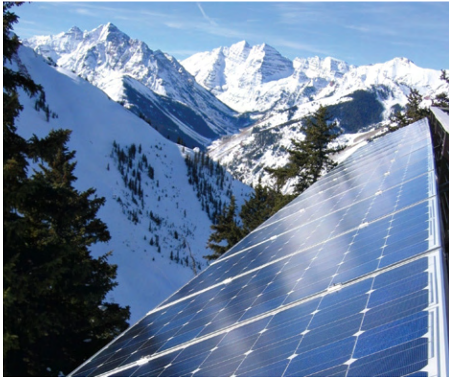
2.4-kW PV system manufactured by GE, installed at 11,000 foot elevation, on the roof of the Highlands Patrol HQ building at the Aspen Mountain Resort in Aspen, CO.
