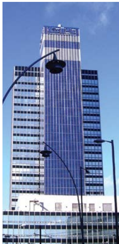
The 25-story CIS Tower in Manchester, UK, is clad in crystalline silicon photovoltaic cells. As thin film technologies mature, applications like this are expected to become much more economical and widespread.
