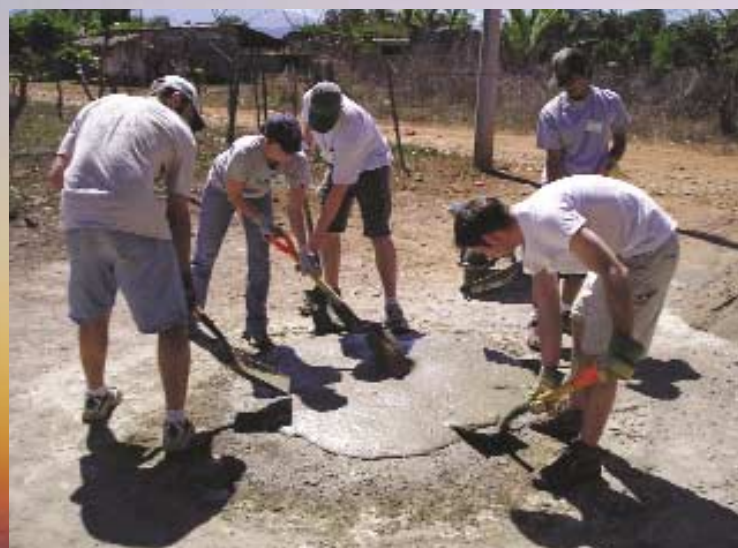
Lacking a mechanical mixer, Eirik, Amy, Steve, Mike and John are mixing concrete with hand tools.
