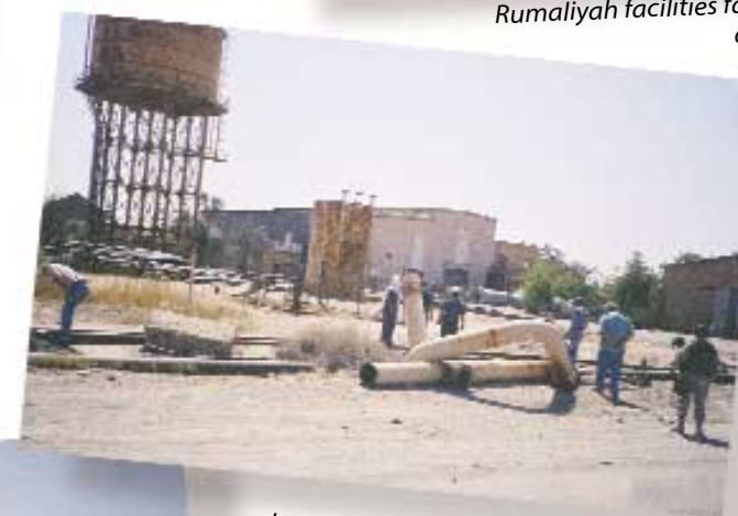
Inspecting South Rumaliyah destroyed pipelines.
