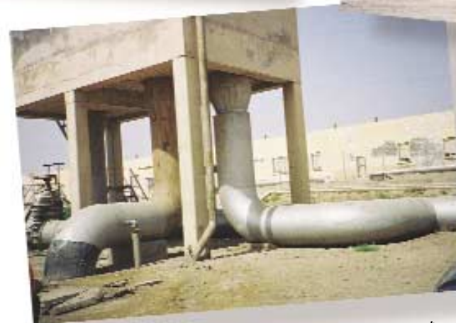
150 million bbl water per year injection system at Garmat Ali plant.
