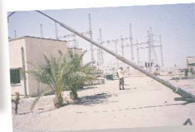
Rumaliyah facilities falling apart after war damage and looting.
