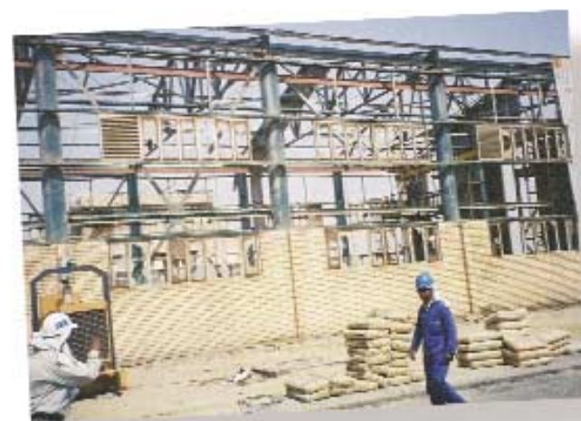
Garmat Ali water plant facilities looted bare (including the roof).
