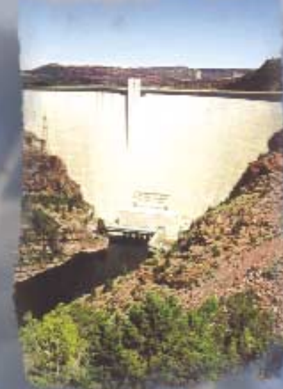
Flaming Gorge Dam in Dutch John, Utah. The EMFI toured the 502-foot-high dam, which houses three 36-MW generators.
