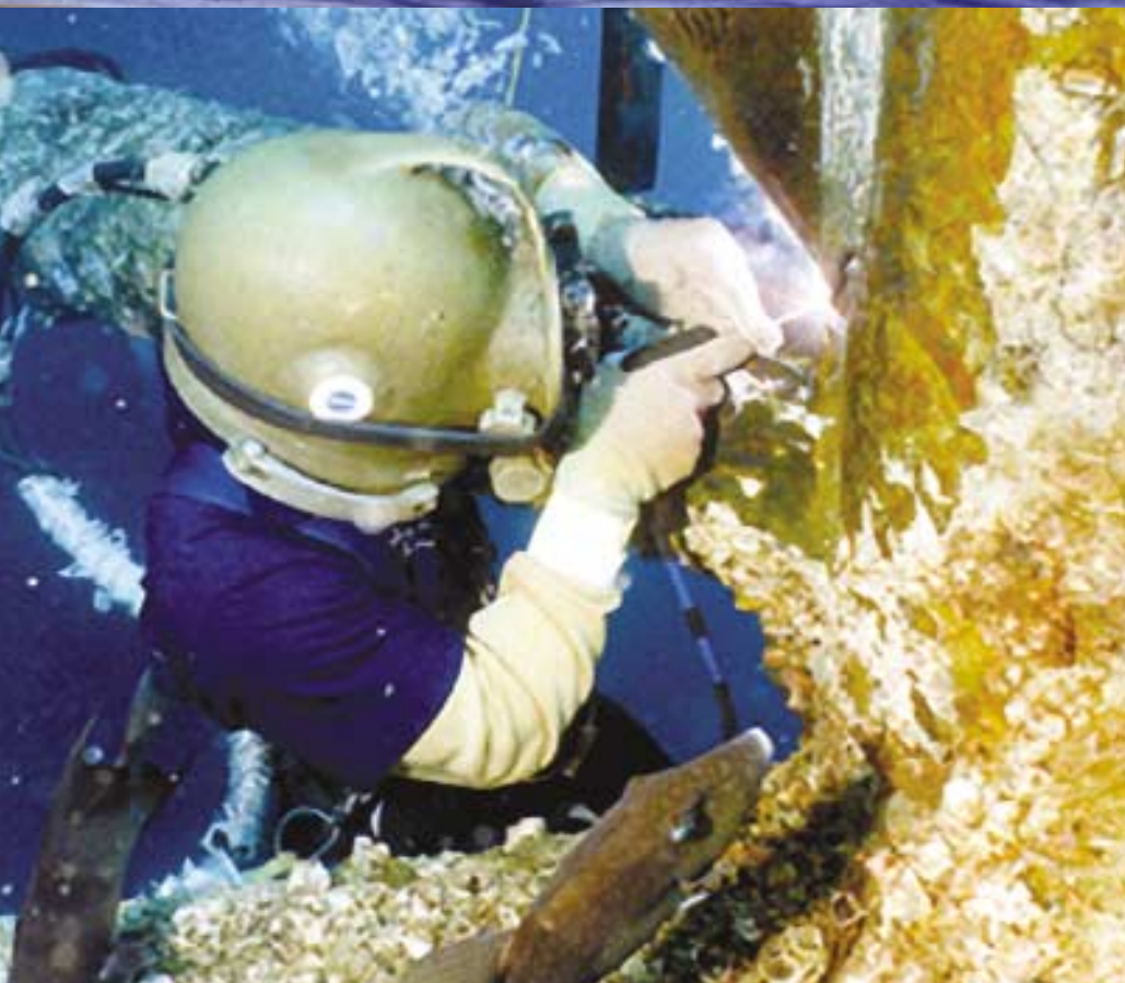
Wet welding is no easy task! (courtesy of Tom Reynolds, Global Divers & Contractors)
