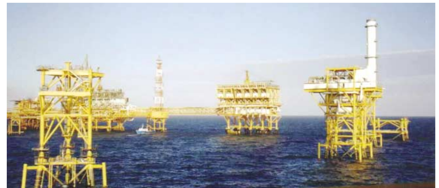
Off-shore platform (courtesy of Ing. Faustino Perez)
