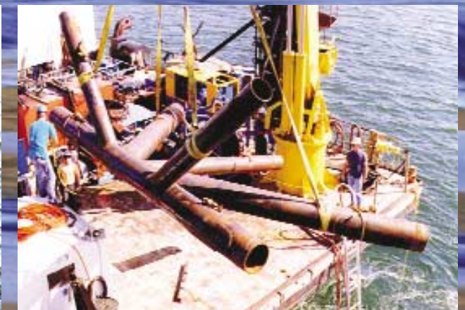
Replacing horizontal K-brace members (courtesy of Tom Reynolds, Global Divers and Contractors)
