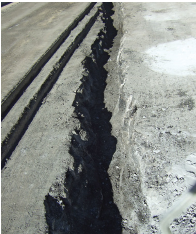
Every year since the 1970s, the eastbound lane has subsided a few inches during springtime snow melt. This fissure was found after asphalt was removed for repairs in summer 2012.
