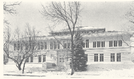
Geophysics Wing, Barlow Hall.
