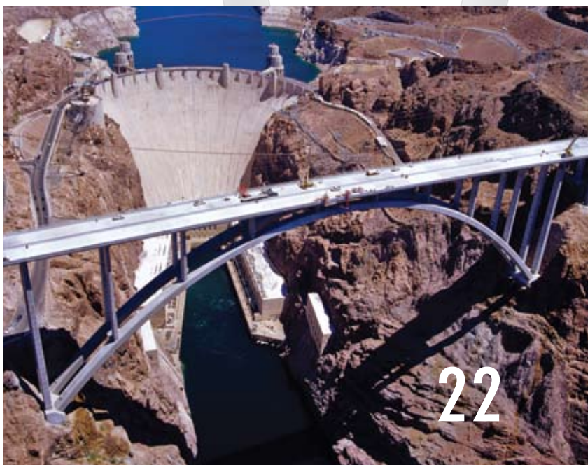
Courtesy of Hoover Dam Bypass Bridge Project
