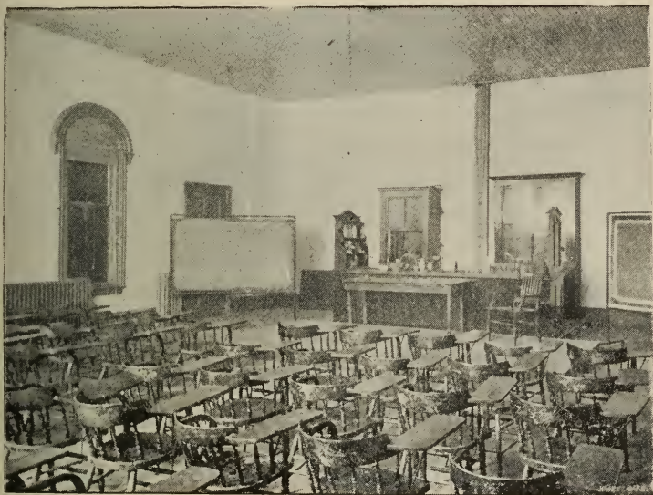
CHEMICAL LECTURE ROOM.
