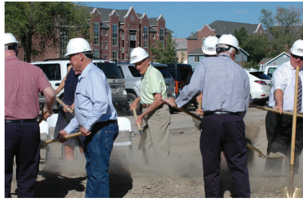
A ceremonial groundbreaking was held September 6, 2016 at 1410 N. Seventh Street for CMU’s newest academic building which will house CMU’s engineering programs and the John McConnell Math & Science Center.
