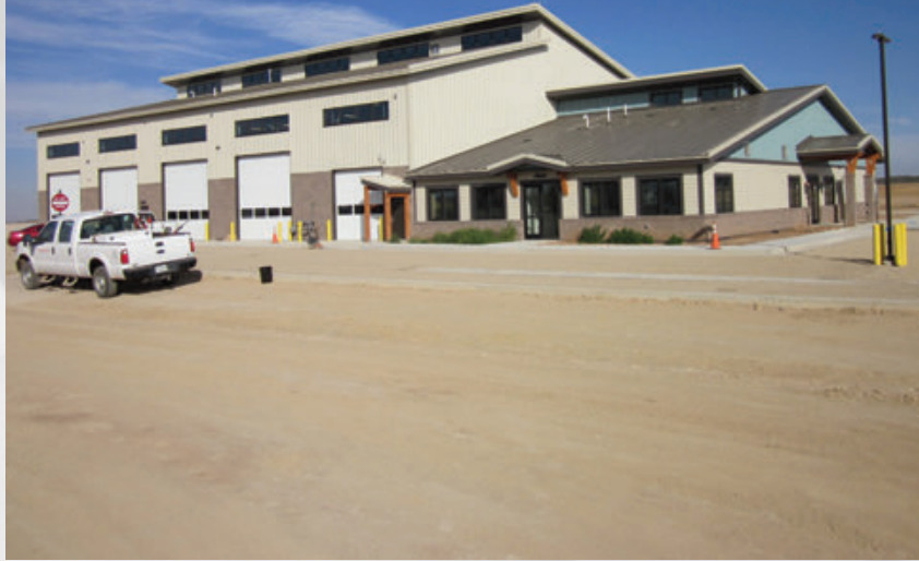
Dolores County New Public Service Center: combination new facility for road and bridge, GIS, and emergency services for county operations
