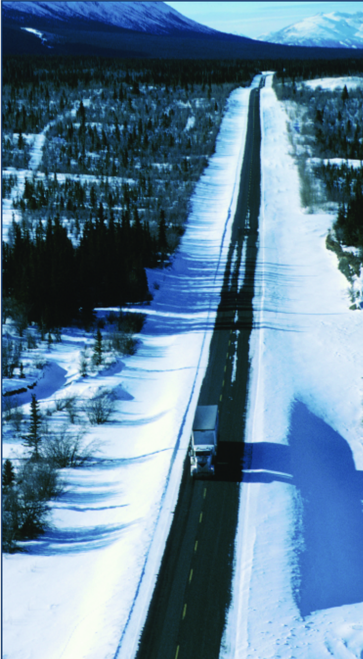
A truck travels the Alaskan Highway through the Canadian Rockies. Permafrost affects buildings, roads, and infrastructure in a variety of Arctic and alpine regions, including communities in Alaska, Canada, Russia, and China. (Courtesy Photos.com)
