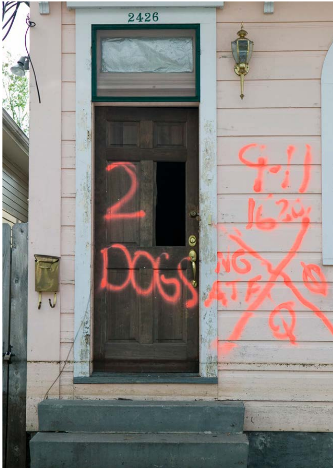
Damage to homes and property in Lower 9th Ward due to Hurricane Katrina. Markings on house were from the Search and Rescue teams searching for survivors following the storm - the date searched, time, who the search party was, survivors found and animals still in the house." © Andrea Booher / FEMA, 2005, New Orleans, Louisiana.
