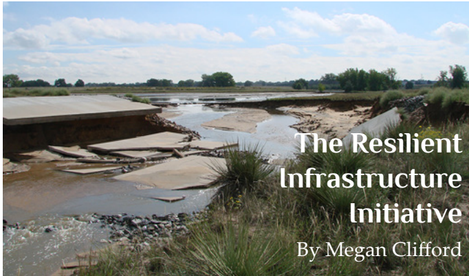
The Havana Pond Dam, City of Denver, Colorado breached and failed on Thursday, Sept. 12, 2013 © USFWS Mountain-Prairie 2013
