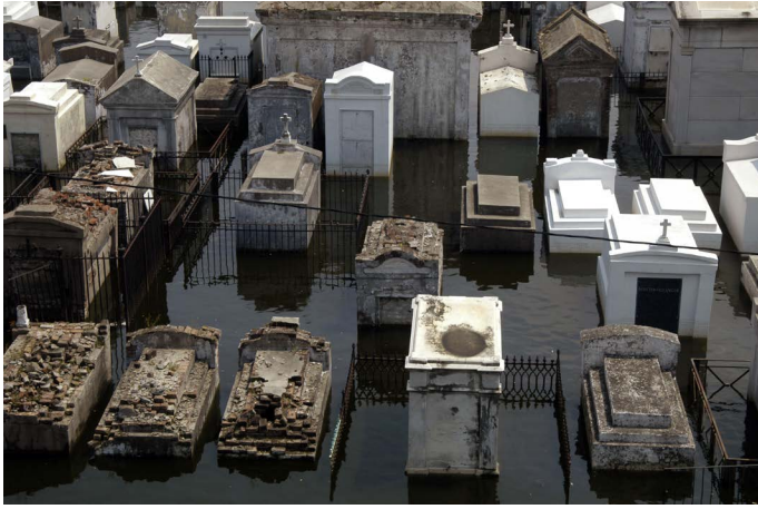
Fig. 2 – Even close up, the damage seems “wet,” but minimal. This is St. Louis No. 1 Cemetery in New Orleans, following the aftermath of Hurricane Katrina in 2005. © FEMA.
