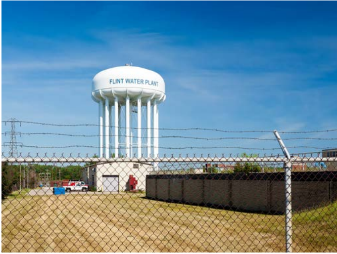
Flint Water Plant © June 2016 George Thomas
