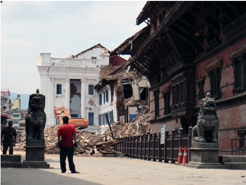
A Nepali soldier stands guard while a man gazes at the severe damage to Basantapur tower and royal palace at Kathmandu's Durbar Square, a UNESCO world heritage site. @ Anne Sanquini
