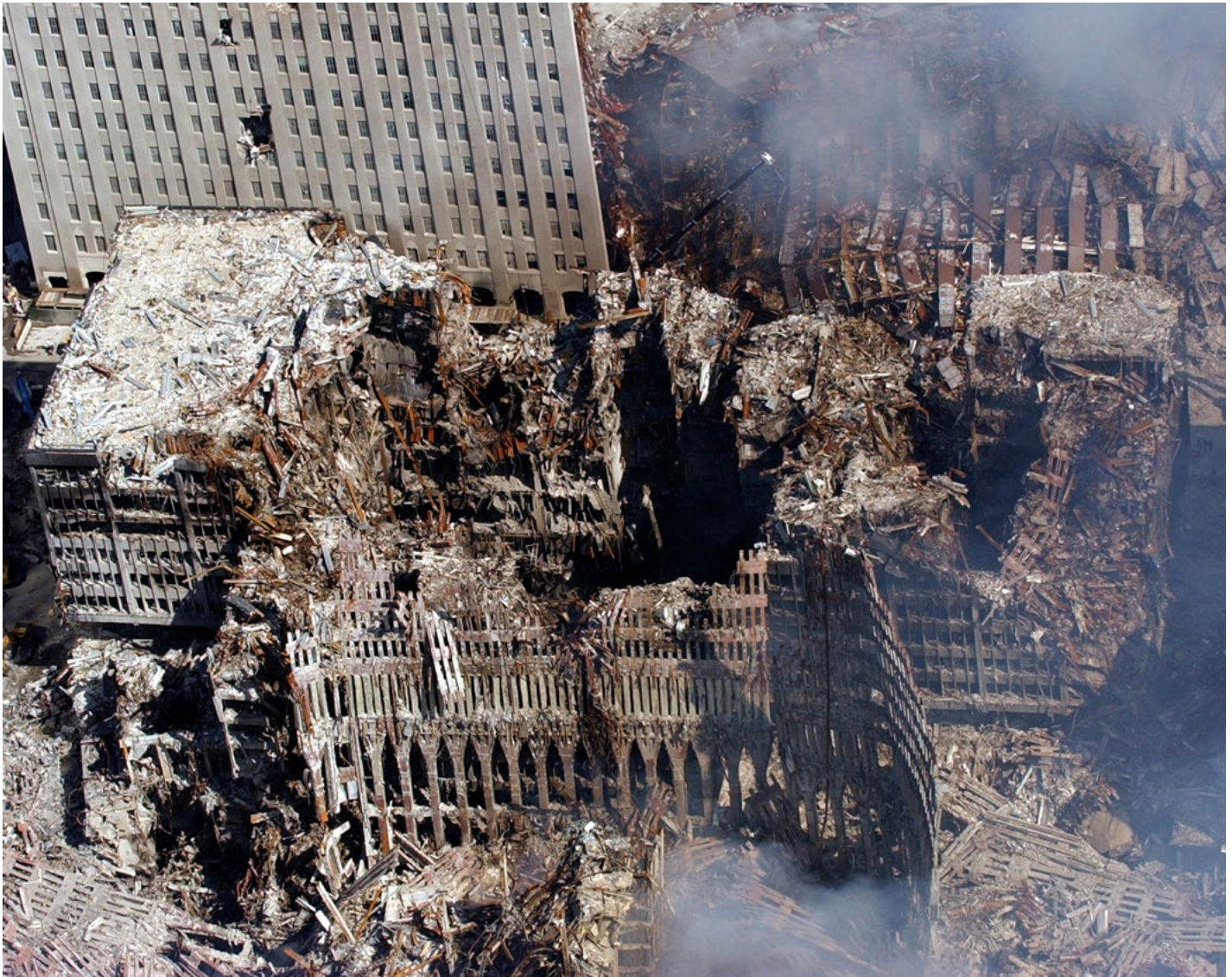
Ground Zero, New York City, N.Y. (Sept. 17, 2001) -- An aerial view shows only a small portion of the scene where the World Trade Center collapsed following the Sept. 11 terrorist attack. Surrounding buildings were heavily damaged by the debris and massive force of the falling twin towers. @ U.S. Navy photo by Chief Photographer's Mate Eric J. Tilford.
