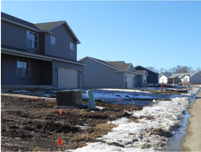
In March 2015, 16 months out from the tornado, Washington's residential areas are over 75% rebuilt. © Rozdilsky (03-07-15).
