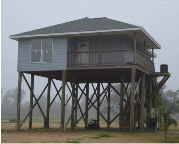
An elevated home outside the southeastern levees. While this structure makes no attempt to minimize the visibility of its elevation, other such pile-supported structures in the area go to great lengths to disguise their elevation through such methods as construction of earthen berms and stage set-like false ground floor walls.
