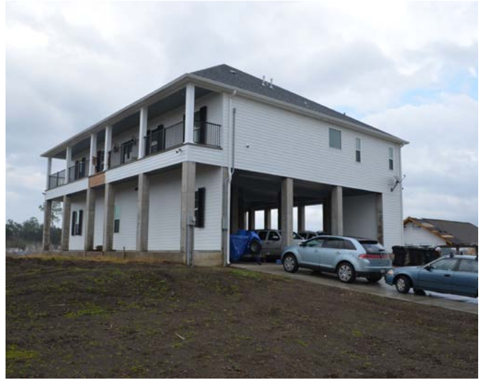
A Braithwaite house rebuilt after flooding from Hurricane Isaac in 2012. Though the house is built nearly twenty feet above the surrounding natural grade, the homeowners opted to built atop an earthen mound and to build a front wall across the uninhabited lower level so as to minimize the appearance of their elevation.
