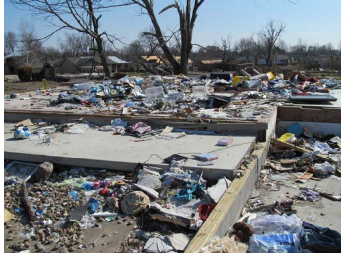
Scenes typical of the residential destruction left in the wake of the tornado. © Rozdilsky (04/05/14).
