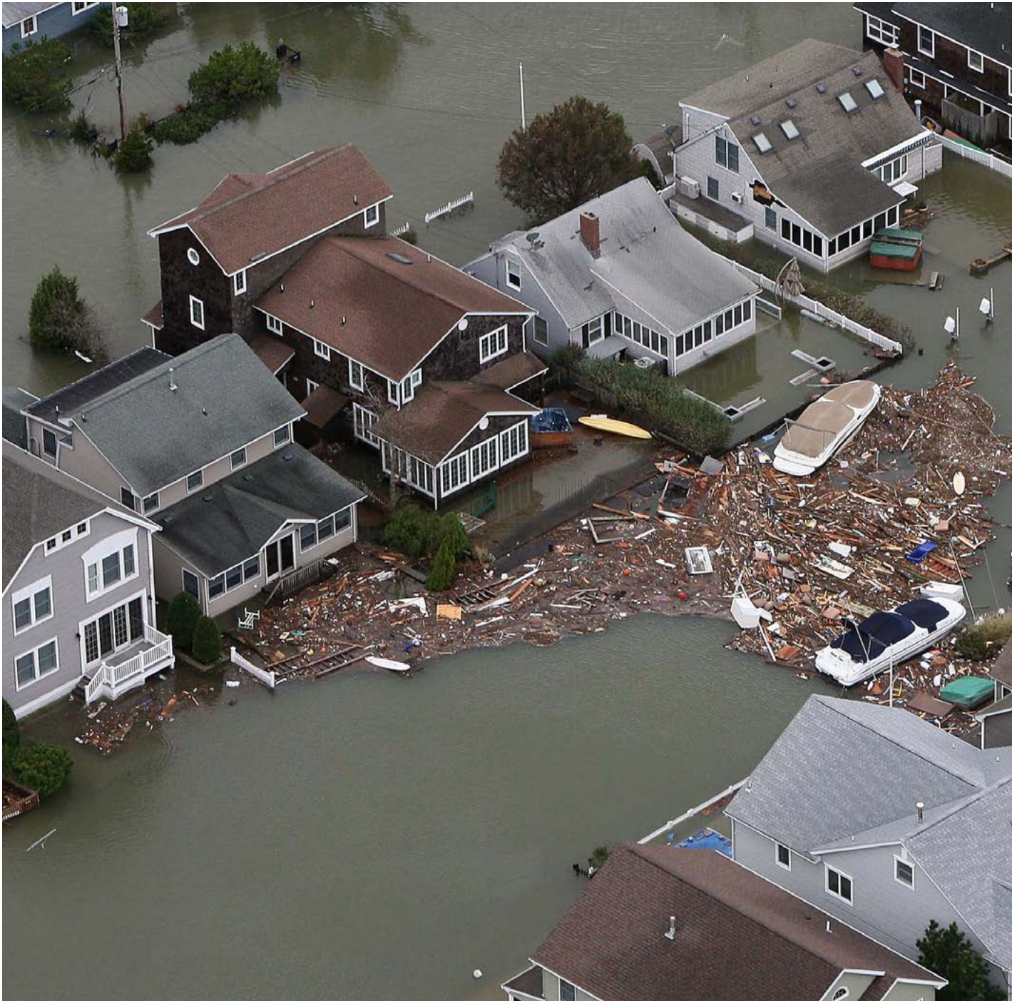
Image 1. Survey of Sandy damage on New Jersey shoreline, October 30, 2012. Source: Courtesy of Tim Larsen, N.J. Governor's Office
