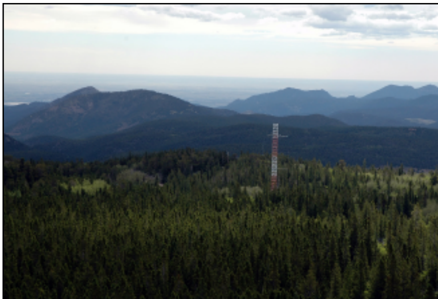
Forty-meter eddy-flux correlation tower near the INSTAAR Mountain Research Station's C1 climate station, erected in the summer of 2004 as part of an NSF Biocomplexity Project headed by Russ Monson (Ecology and Evolutionary Biology and CIRES) and Dave Schimel (NCAR) to study CO 2 uptake by forest canopies in complex mountain terrain, near Ward, Colorado, September 2004. Photo: W. Bowman (INSTAAR).
