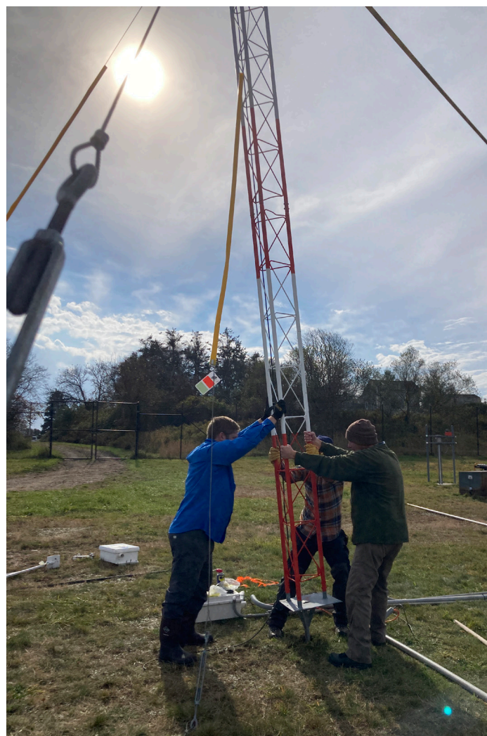
Wind Forecast Improvement Project (WFIP-3) researchers raise a tower on Block Island for this collaborative project, which aims to improve weather forecasting in the area, especially for offshore wind farms. Photo: Laura Bianco/ CIESRDS
