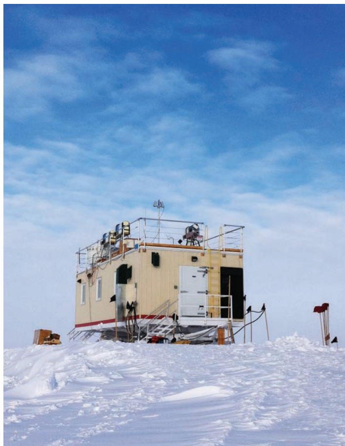
The Mobile Science Facility at Summit, Greenland, houses the National Science Foundation–sponsored Integrated Characterization of Energy, Clouds, Atmospheric state, and Precipitation at Summit (ICECAPS) Project.
