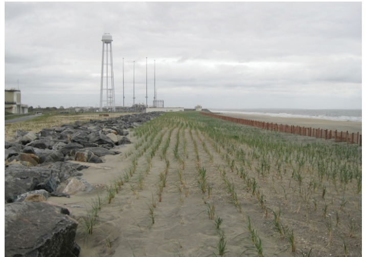
The NASA Wallops Flight Facility launch range along Virginia's eastern shore. In the distance is a launch pad recently used to launch an Antares rocket. In the foreground are storm-mitigation measures put in place after Hurricane Sandy. The Atlantic Ocean is on the right.
