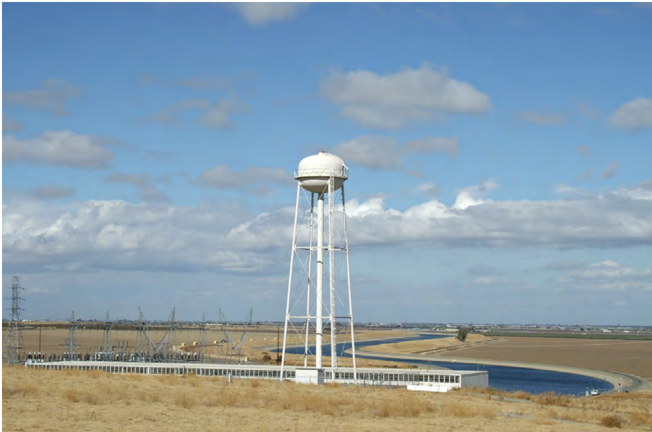
Water-pumping station near Los Banos, Calif.
