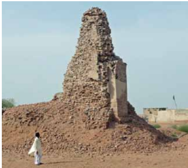
The “Thul” at Mansurah in 2008. This masonry tower is all that remains of fortified town of Mansurah, the ancient capital of Sindh province that was destroyed by an earthquake c. 980 AD. In 19th century archaeological excavations, skeletons were found crushed by bricks. Recent excavations revealed four massive bronze door knockers buried deep beneath the ruins of the largest building, objects that had escaped looting in the past millennium, which would surely have been removed if the city had, instead of being shaken by an earthquake, been sacked by an invading army.
