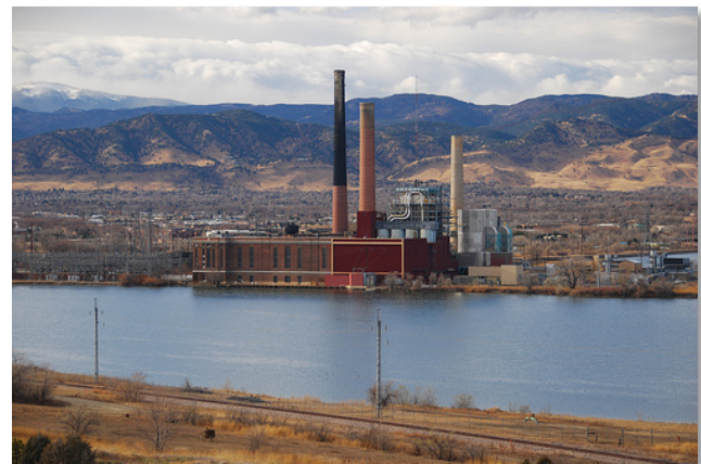
Figure 3. Valmont power plant, Boulder, Colorado. Photo courtesy Let Ideas Compete.
