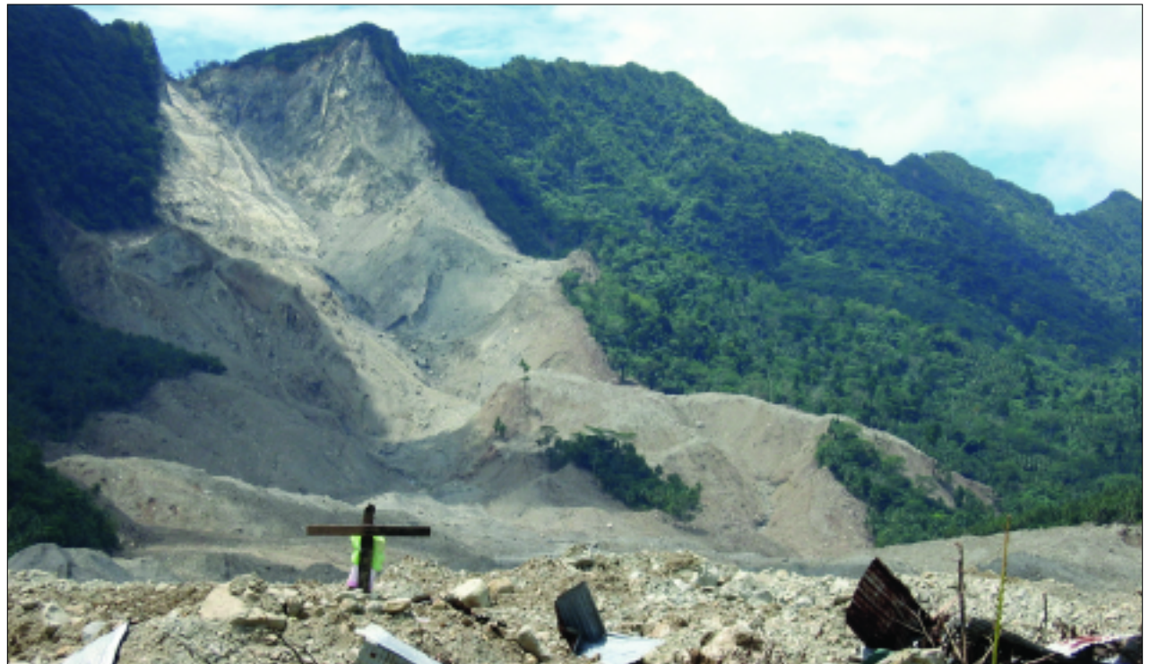
Debris from the February 17, 2006, landslide that buried Guinsaugon shows the effect of tectonic weakening. The landslide occurred along a fault line, where tectonic movement grinds and crushes the rock. This ground-up rock and soil on the mountainside had become more prone to landslides, especially after several days of rain. (Courtesy Stephen Evans)
