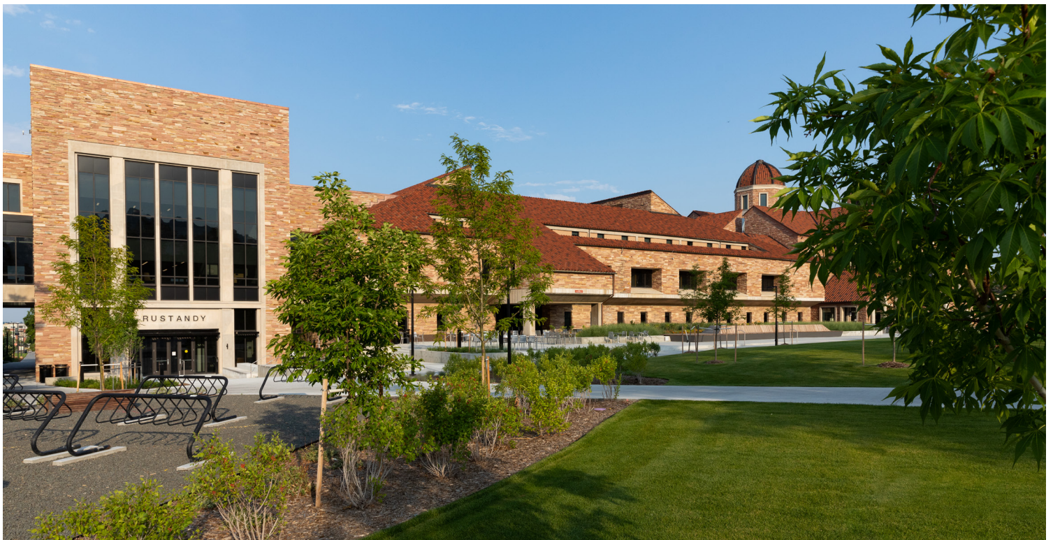
Rustandy addition at the Leeds School of Business, University of Colorado Boulder.
