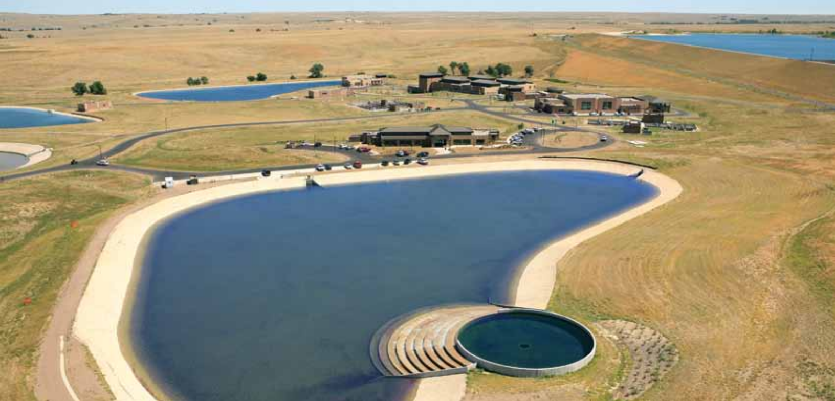
Binney Water Purification Facility, part of the Prairie Waters system
