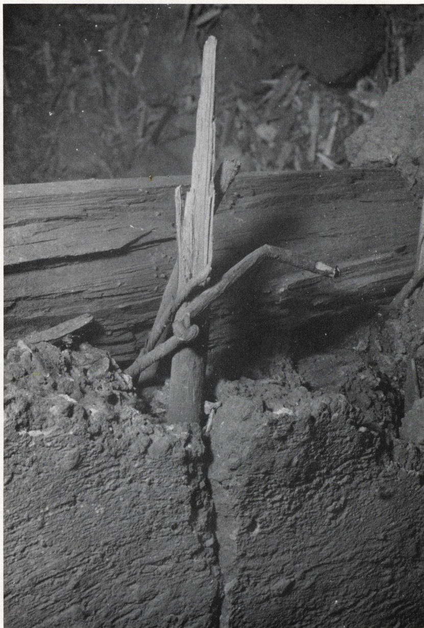
Corral Cave. Detail of post-and-mud wall. Note the willow binding used to tie the horizontal sticks to the vertical posts.
