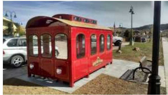
Figure 12: Cripple Creek Bus Shelters
