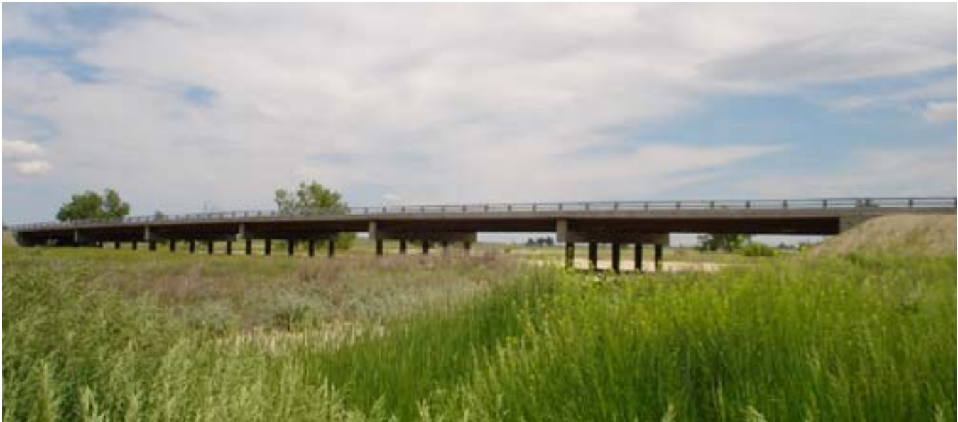
CDOT's first simple made continuous steel bridge, completed in 2006, crosses Box Elder Creek on U.S. 36
