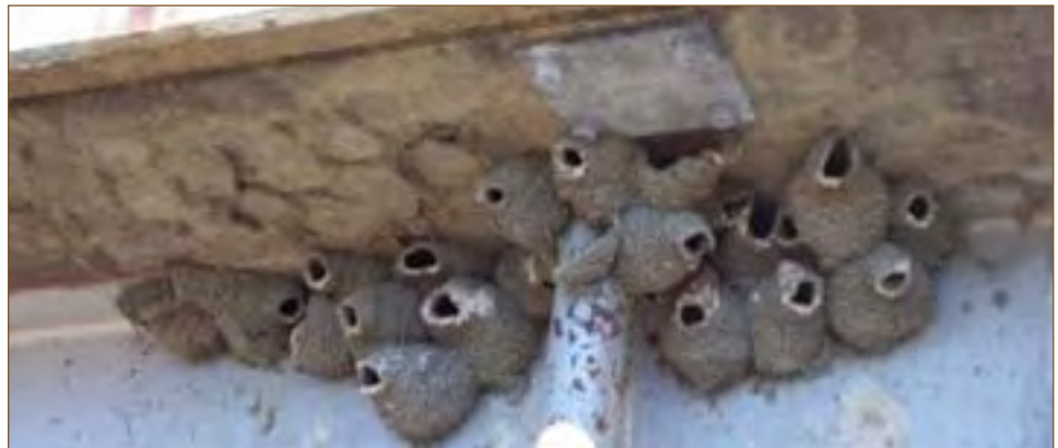
Swallow nests under a bridge deck
