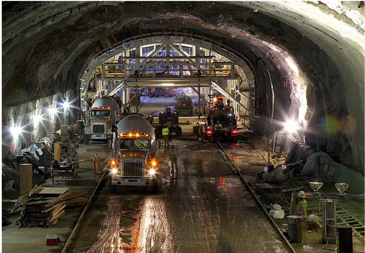
Twin Tunnels under Construction
