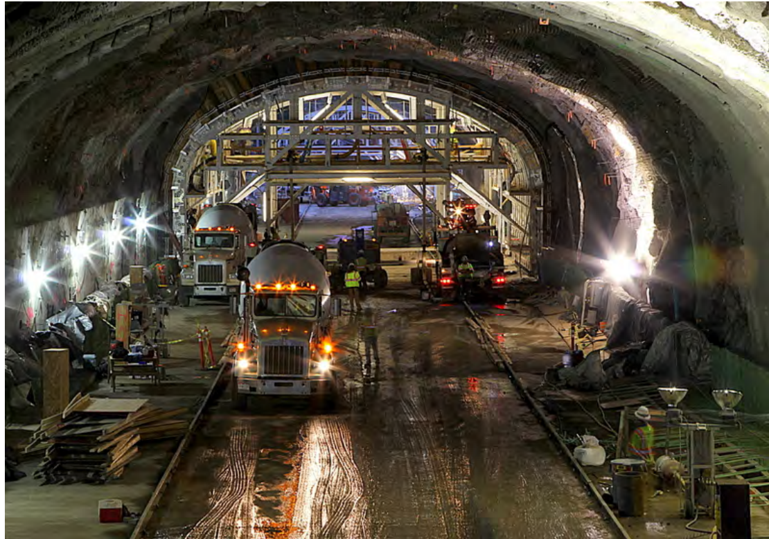
Twin Tunnels under Construction
