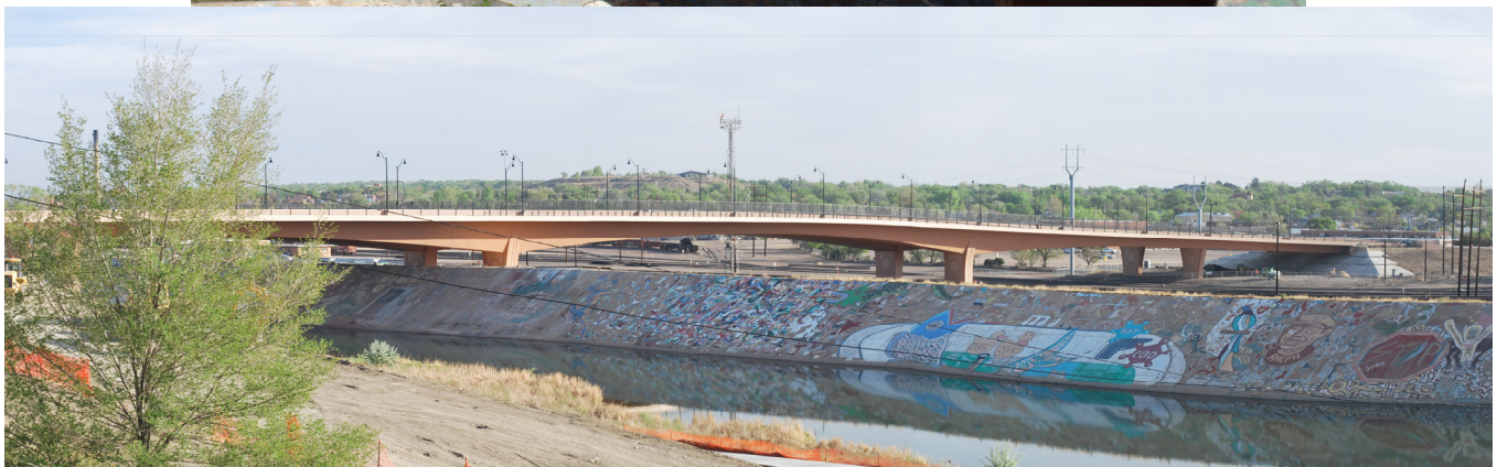
Award Winning 4 th Street Bridge, Pueblo; Longest Bridge Span on the Colorado State Highway System
