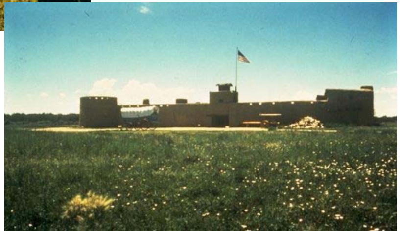
Bent's Old Fort - Santa Fe Trail Byway - U.S. 50 (E of La Junta)
