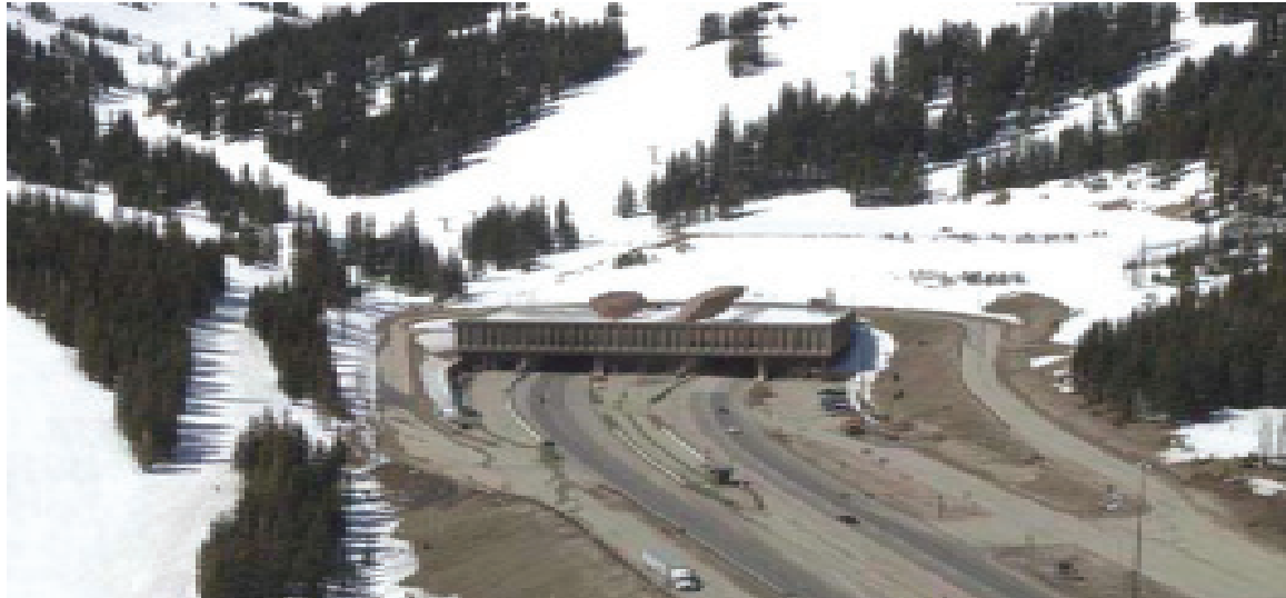
Eisenhower / Johnson Memorial Tunnels – Interstate 70 – Continental Divide
