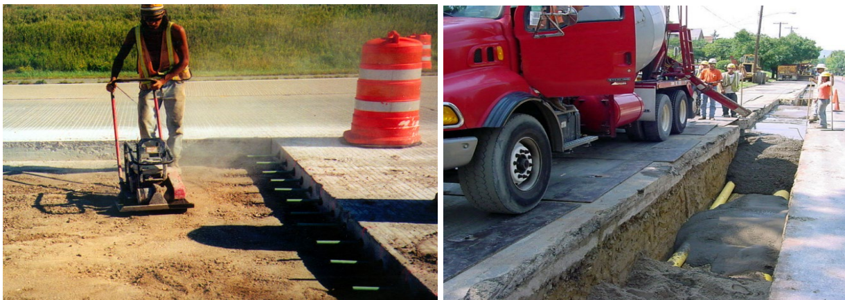
Figure 10.10 Photos of Compaction of Subbase and Flowfill Placement
