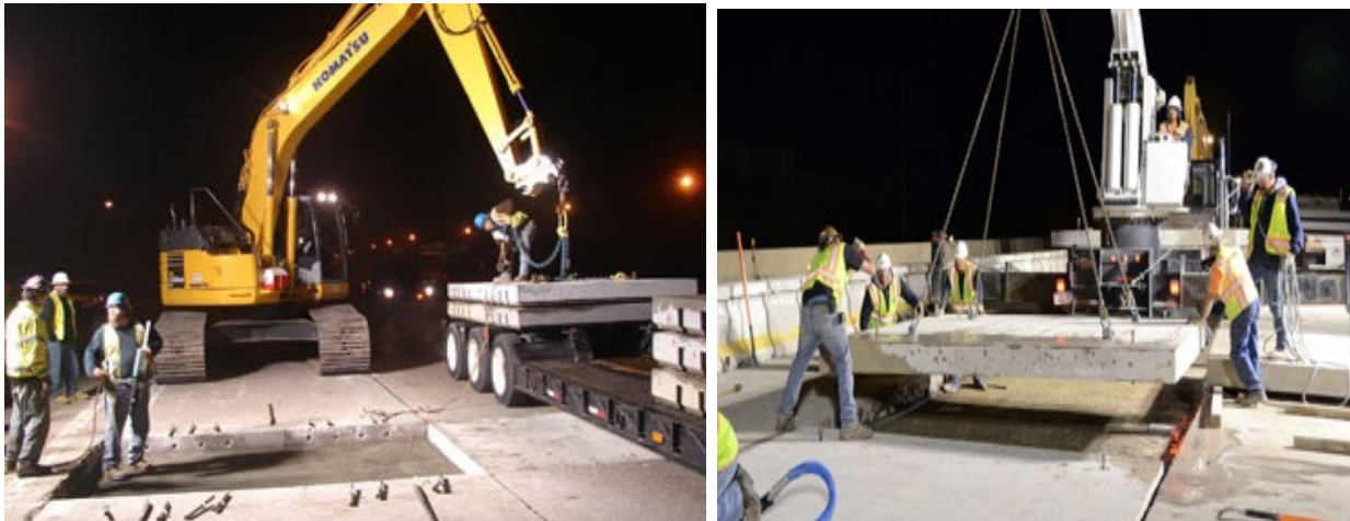
Figure 10.13 Photos of Precast Concrete Panel Repair
