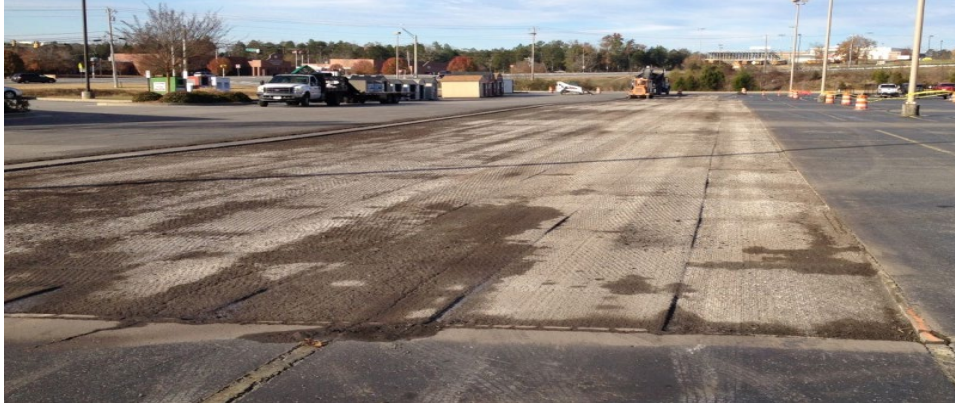
Figure 8.8 Photo of Asphalt After Milling
