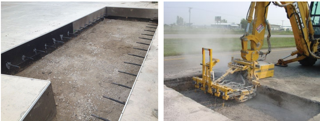
Figure 10.8 Photos of Full Depth Concrete Repair
