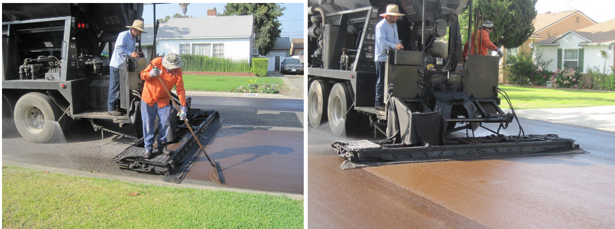
Figure 8.41 Photo Showing the Placing of a Slurry Seal
