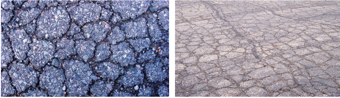
Figure 8.3 Photos of Alligator (Fatigue) Cracking
