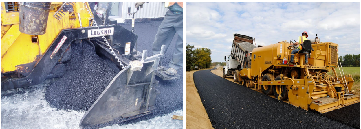
Figure 8.44 Photos of Cold Mix Paving
