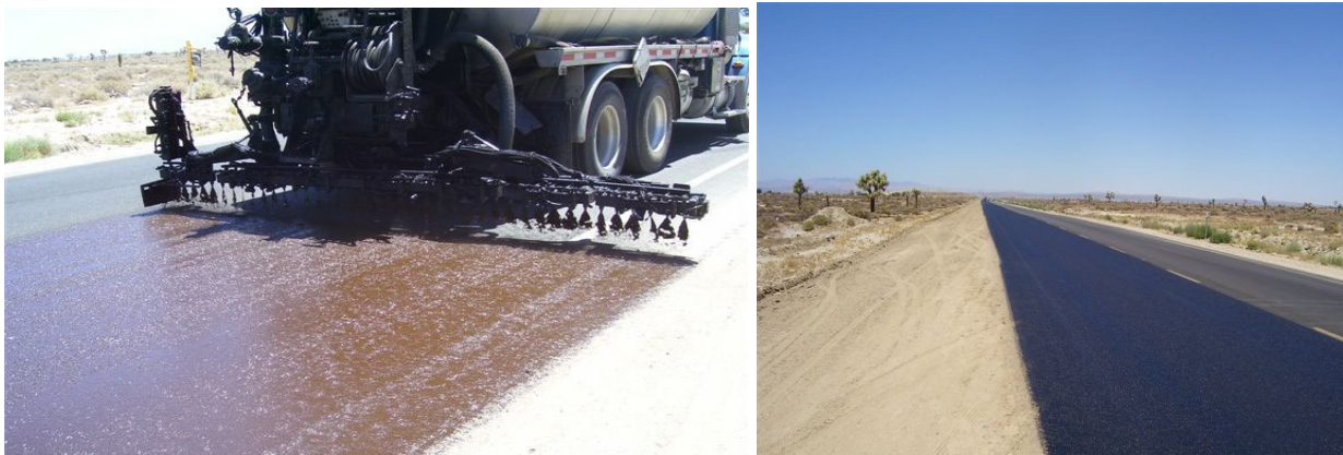
Figure 8.45 Photos Showing the Placing of a Fog Coat and the Final Result
