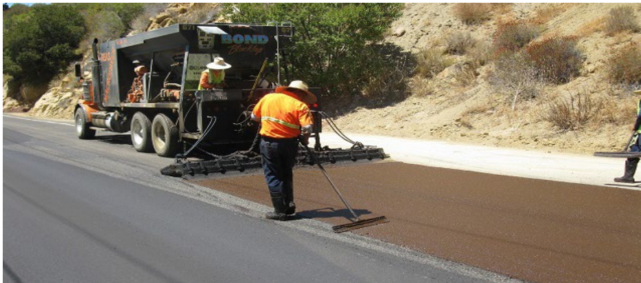
Figure 8.28 Photo Showing Micro-Surfacing
