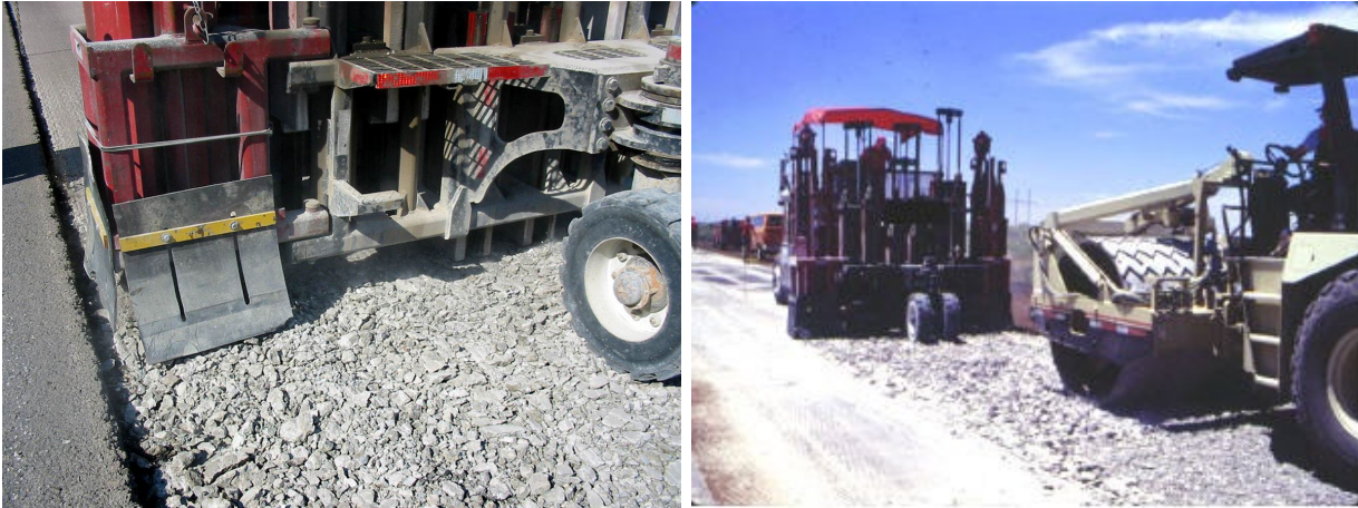
Figure 8.35 Photos of the Rubbilization Initial Operation
