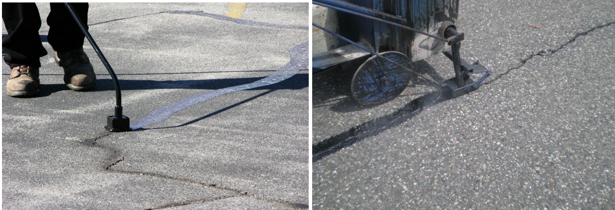
Figure 8.43 Photos Showing Crack Sealing
