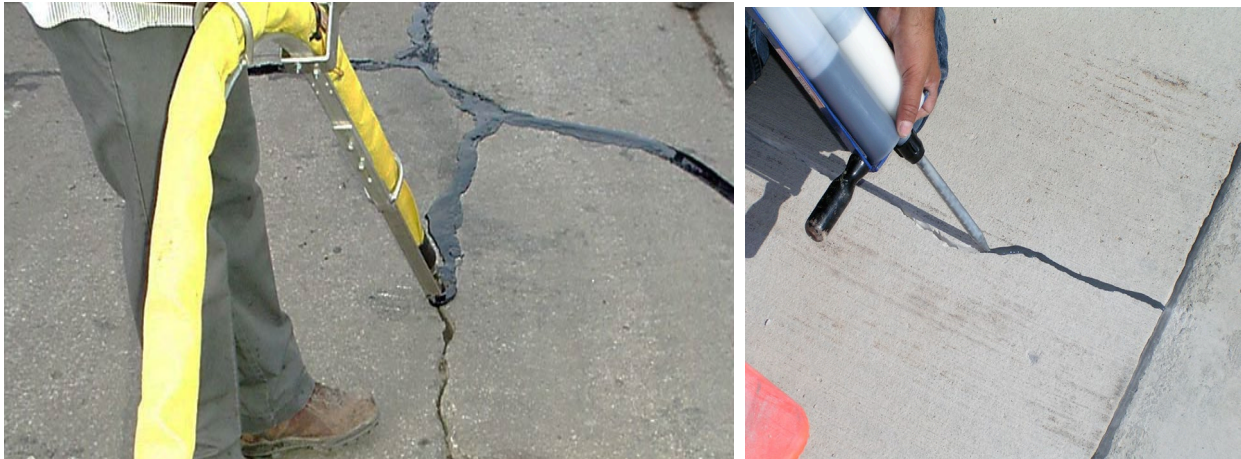
Figure 10.5 Photos of Crack Sealing
