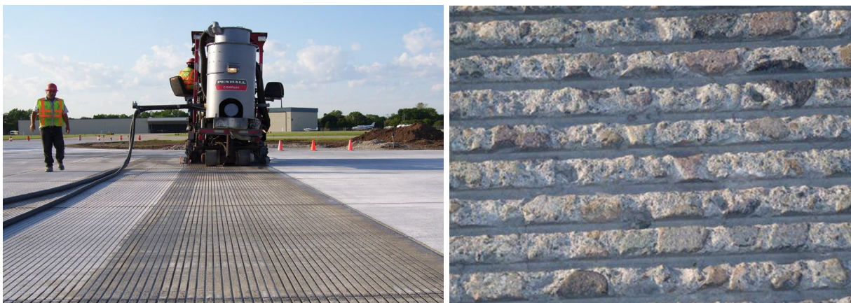
Figure 10.2 Photos of Diamond Grinding and Grooving
