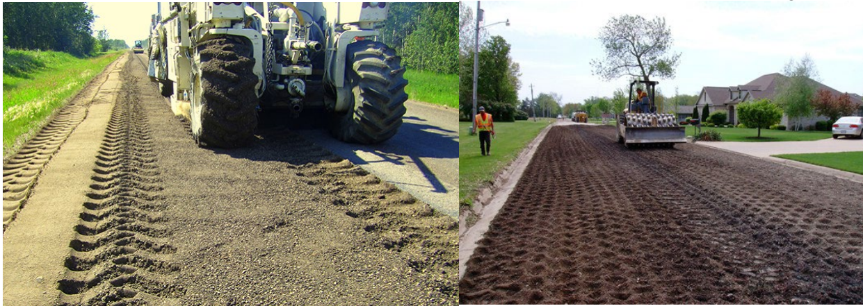
Figure 5.8 Photos of Full Depth Asphalt Reclaimed Base
