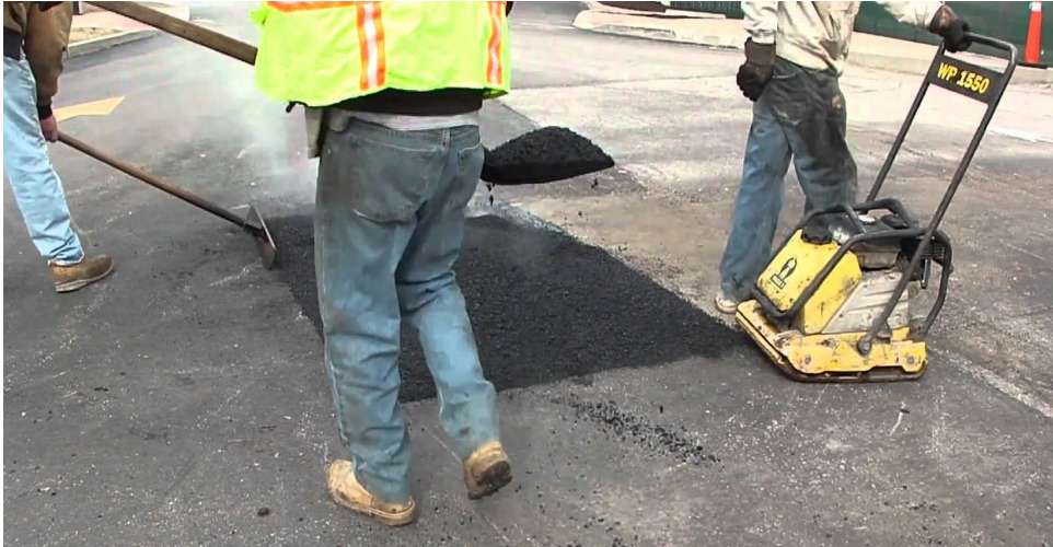
Figure 8.50 Photo of Manual Skin Patching
