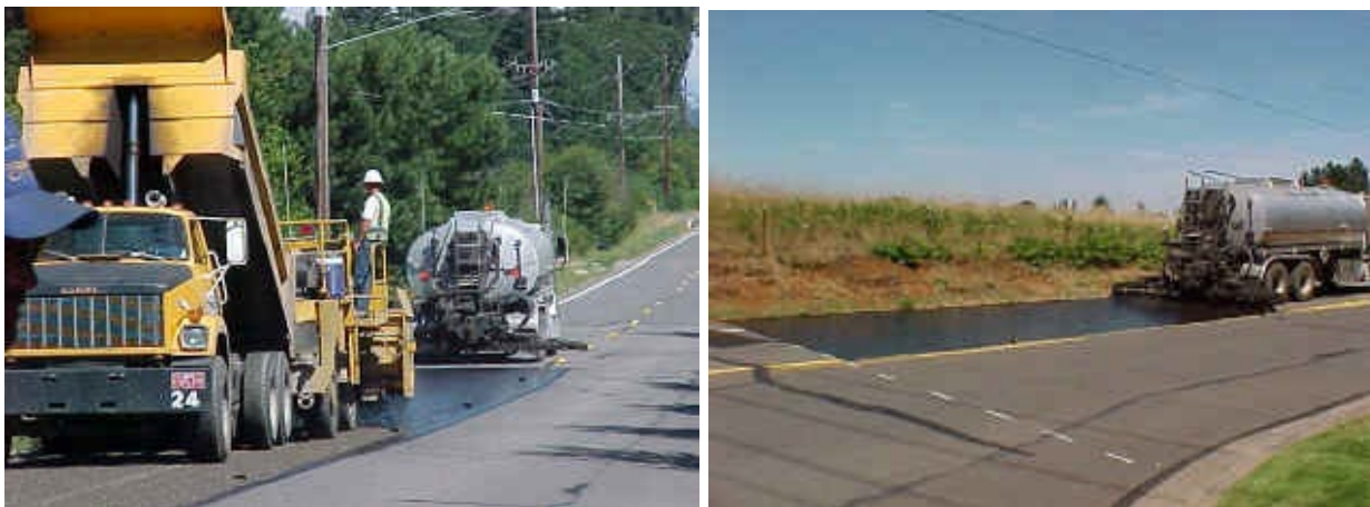
Figure 8.40 Photos Show a Cape Seal Where a Chip Seal is Applied, Cures, and After A Month a Slurry Seal is Applied
