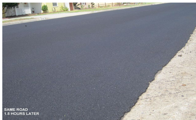
Figure 8.42 Photo Showing a Slurry Seal 1.5 Hours After Placement
