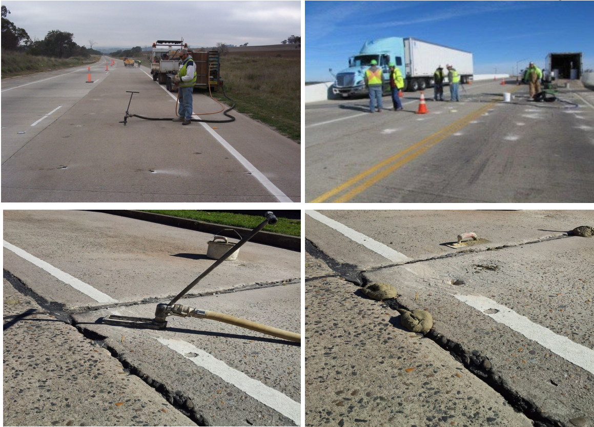
Figure 10.22 Photos of Slabjacking
