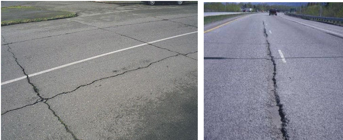
Figure 8.4 Photos of Longitudinal and Transverse Cracking
