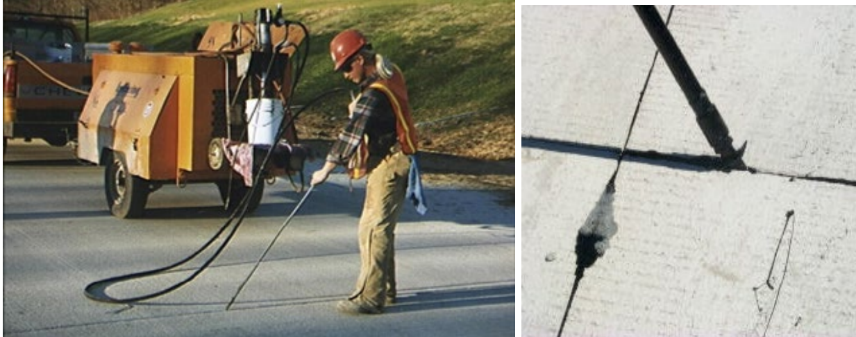
Figure 10.6 Photos of Concrete Joint Resealing
