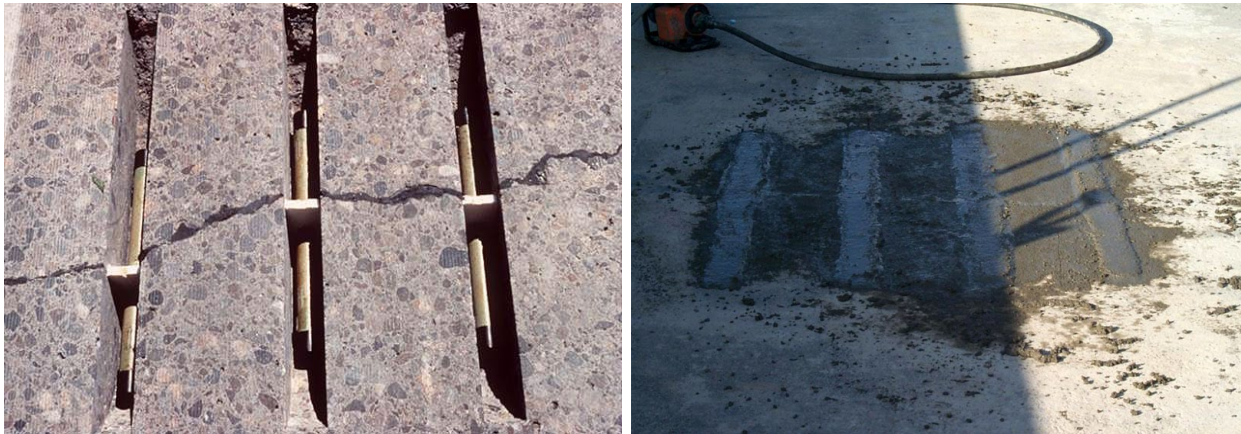
Figure 10.18 Photos of Slot Stitching
