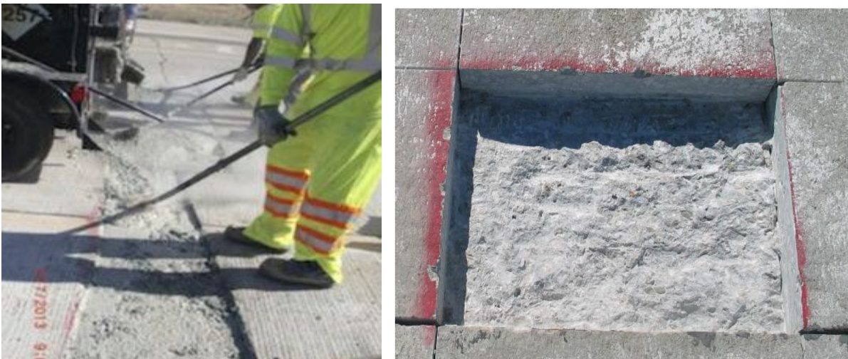
Figure 10.7 Photos of Partial Depth Concrete Repair
