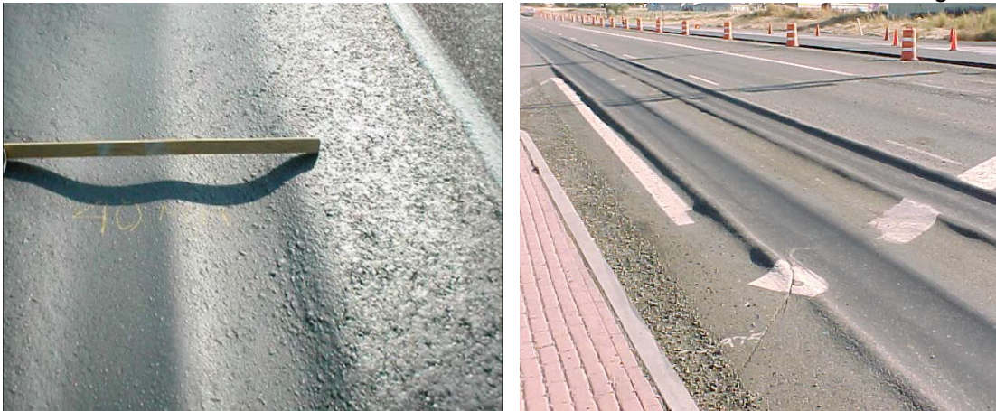
Figure 8.5 Photos of Rutting
