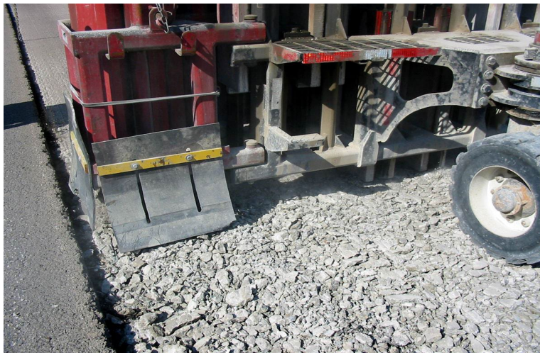
Figure 5.10 Photo of Rigid Pavement Being Rubblized
