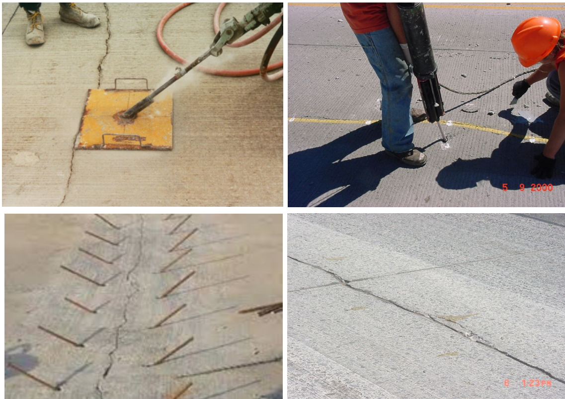
Figure 10.17 Photos of Cross Stitching
