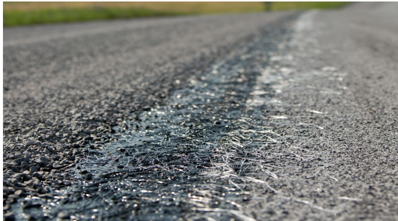
Figure 8.49 Photo Showing a Stress Absorbing Membrane
