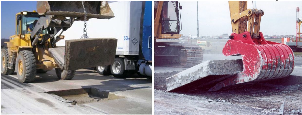
Figure 10.9 Photos of Concrete Slab Removal
