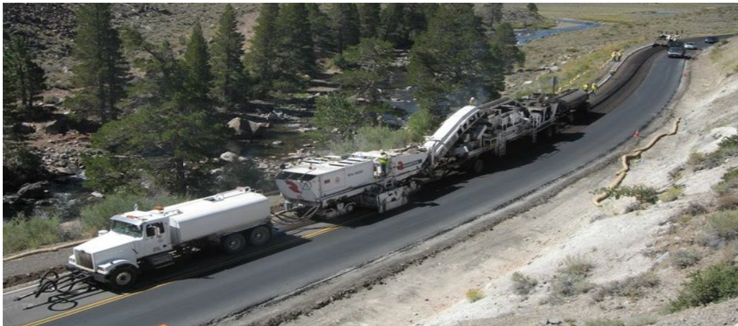
Figure 8.47 Photo Showing A Cold In-Place Recycling Operation
