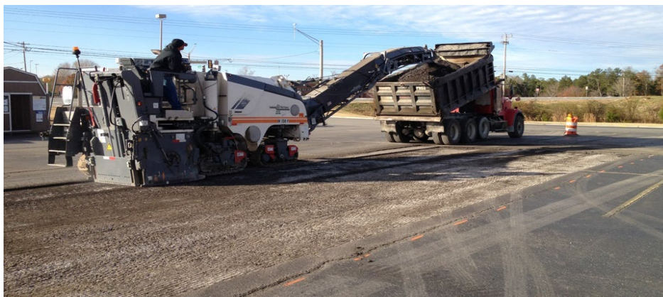
Figure 8.7 Photo of Milling of Old Asphalt
