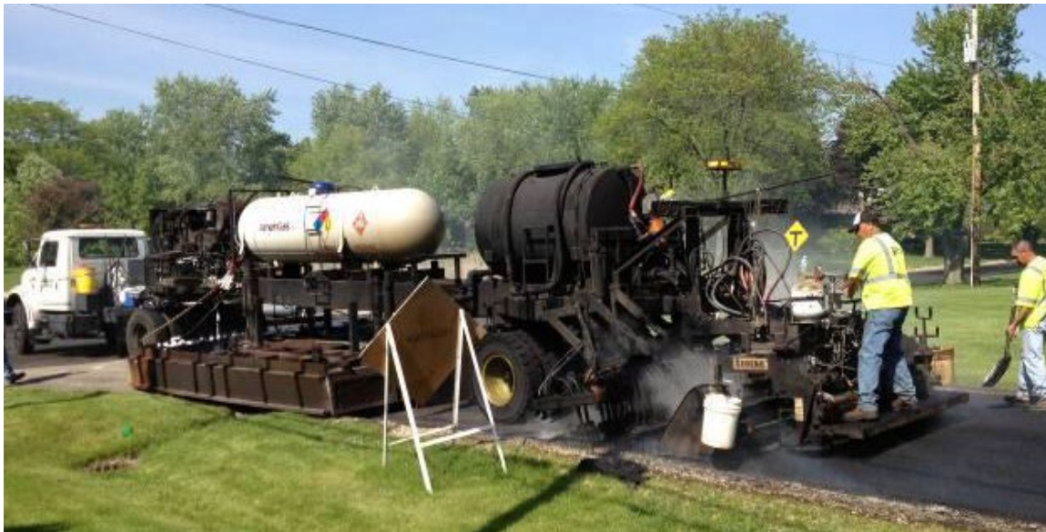
Figure 8.14 Photo of Heating Scarifying Equipment (Initial Operation)
