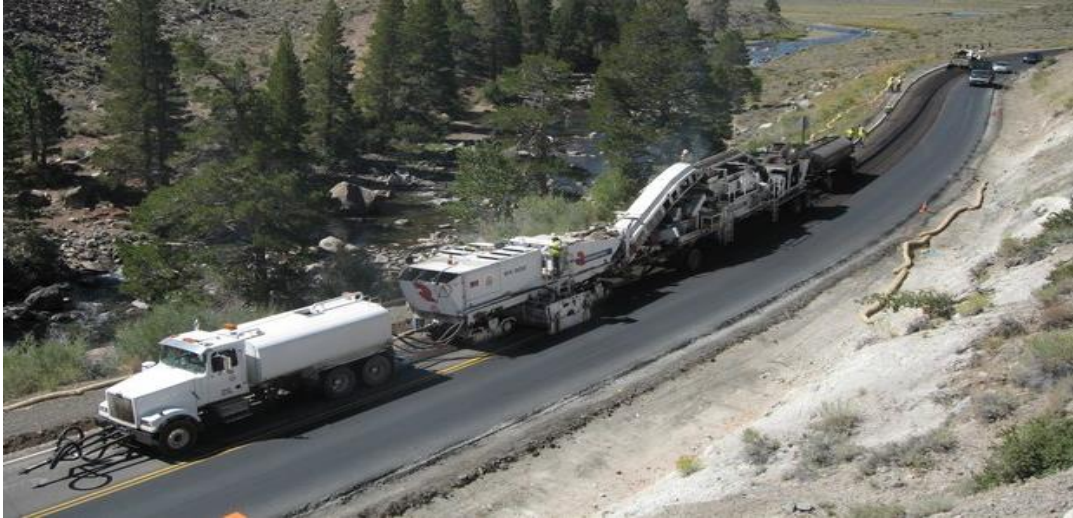
Figure 8.46 Photo Showing A Cold In-Place Recycling Operation
