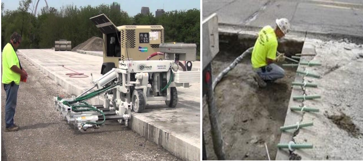
Figure 10.12 Photos of Tie Bar Installation During Concrete Repair
