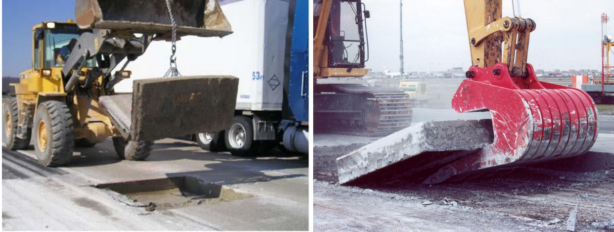
Figure 10.9 Photos of Concrete Slab Removal
