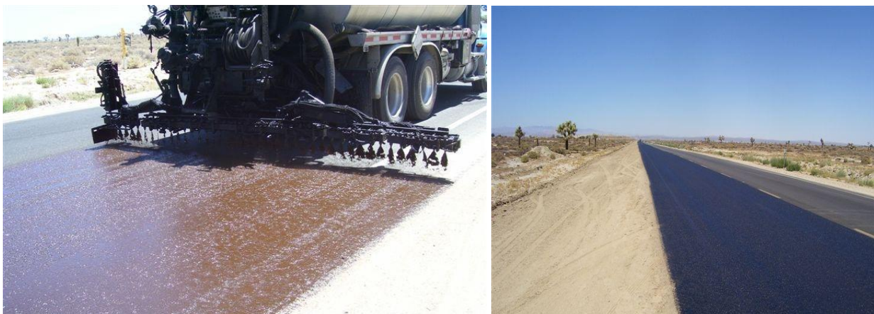
Figure 8.44 Photos Showing the Placing of a Fog Coat and the Final Result
