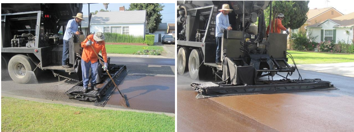
Figure 8.40 Photo Showing the Placing of a Slurry Seal
