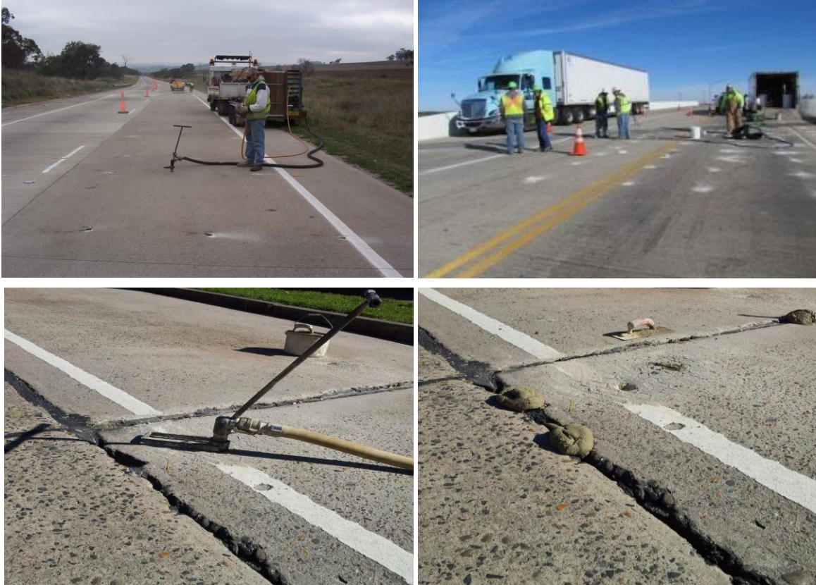
Figure 10.22 Photos of Slabjacking
