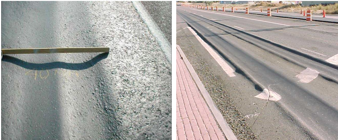
Figure 8.5 Photos of Rutting
