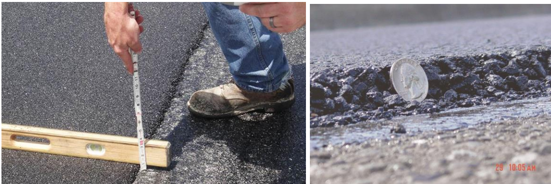
Figure 8.47 Photos of Ultra-Thin Asphalt Overlays
