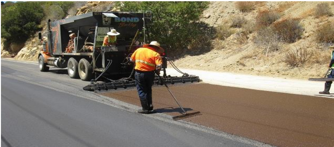
Figure 8.28 Photo Showing Micro-Surfacing
