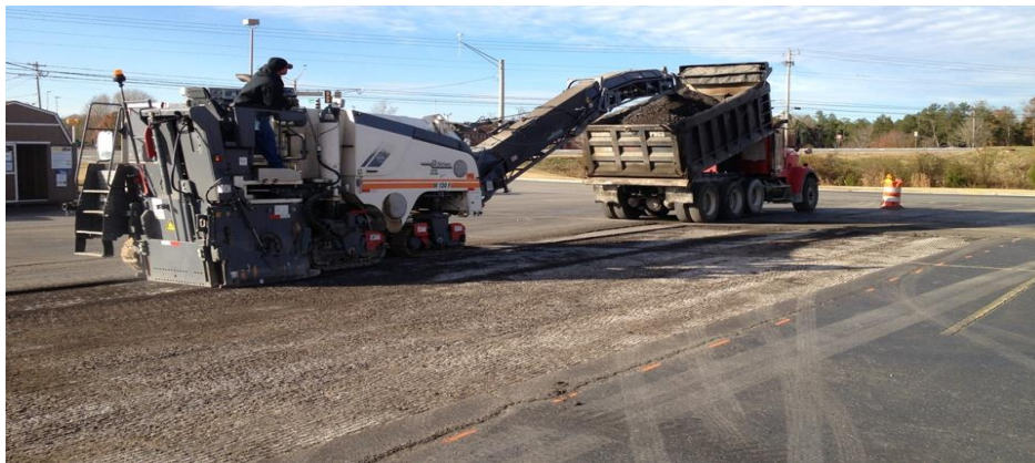
Figure 8.7 Photo of Milling of Old Asphalt
