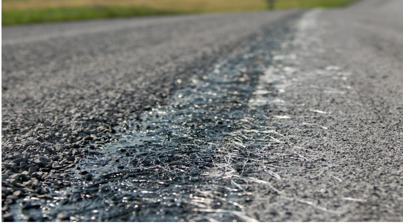
Figure 8.48 Photo Showing a Stress Absorbing Membrane
