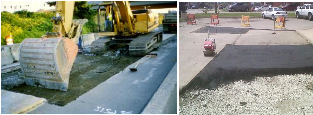
Figure 8.45 Photos Showing Various Stages of Full Depth Replacement Patching
