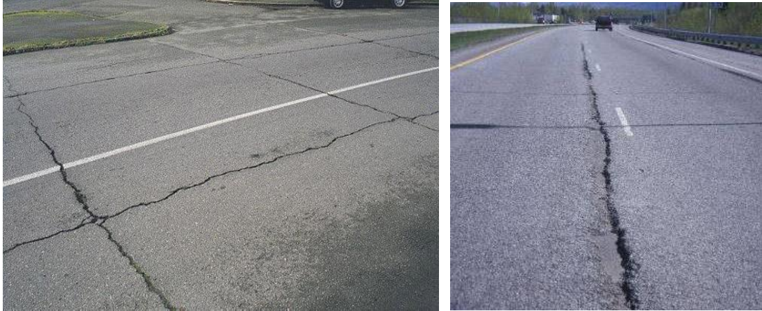
Figure 8.4 Photos of Longitudinal and Transverse Cracking
