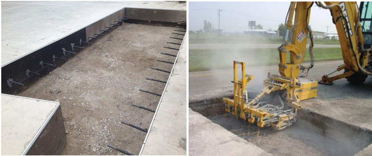
Figure 10.8 Photos of Full Depth Concrete Repair
