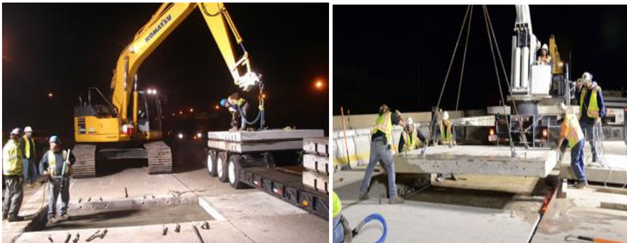
Figure 10.13 Photos of Precast Concrete Panel Repair
