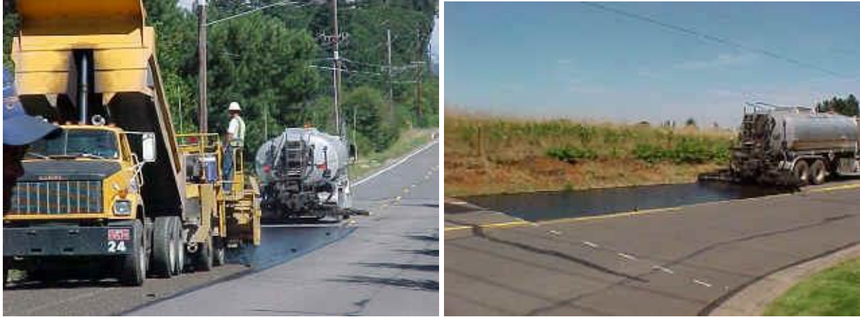
Figure 8.39 Photos Show a Cape Seal Where a Chip Seal is Applied, Cures, and After A Month a Slurry Seal is Applied
