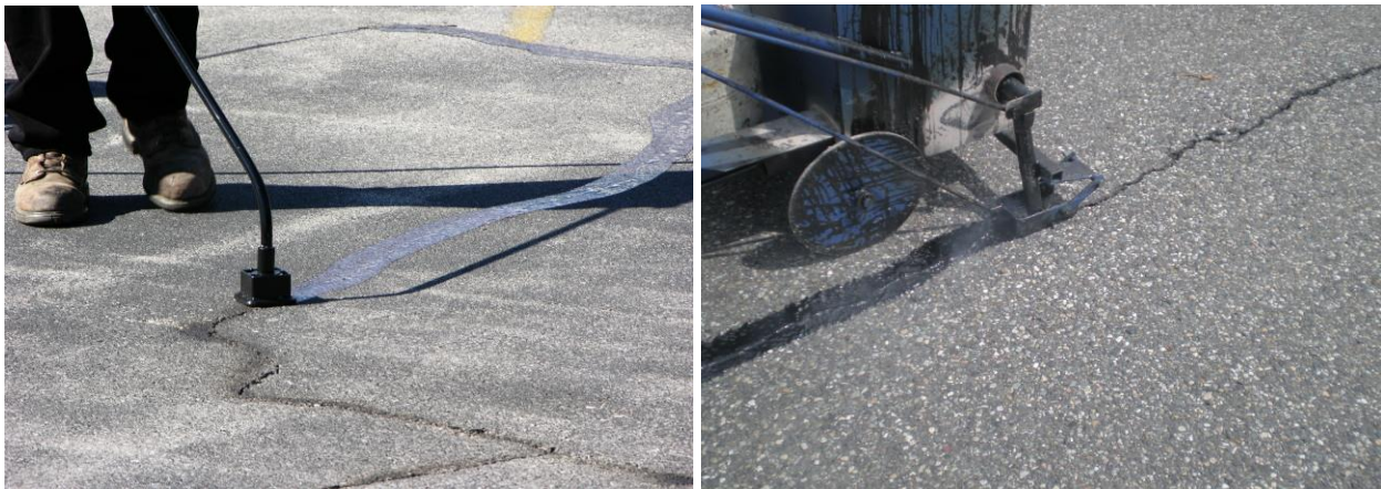
Figure 8.42 Photos Showing Crack Sealing
