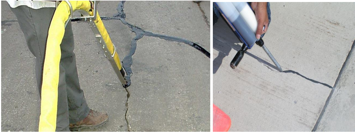
Figure 10.5 Photos of Crack Sealing
