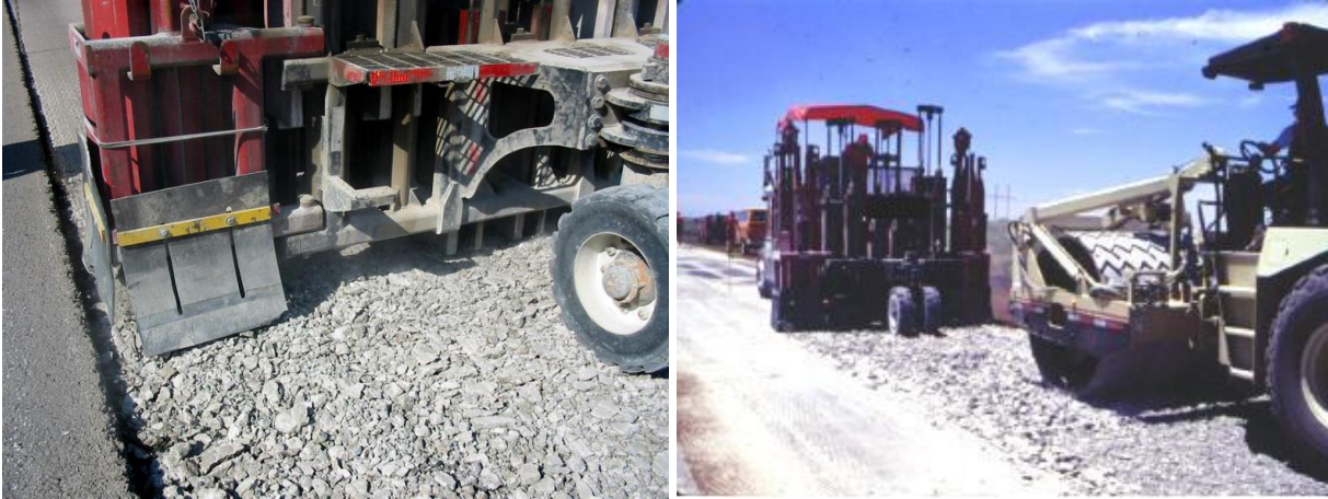
Figure 8.35 Photos of the Rubbilization Initial Operation
