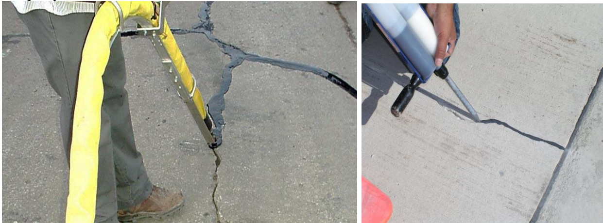
Figure 10.5 Photos of Crack Sealing
