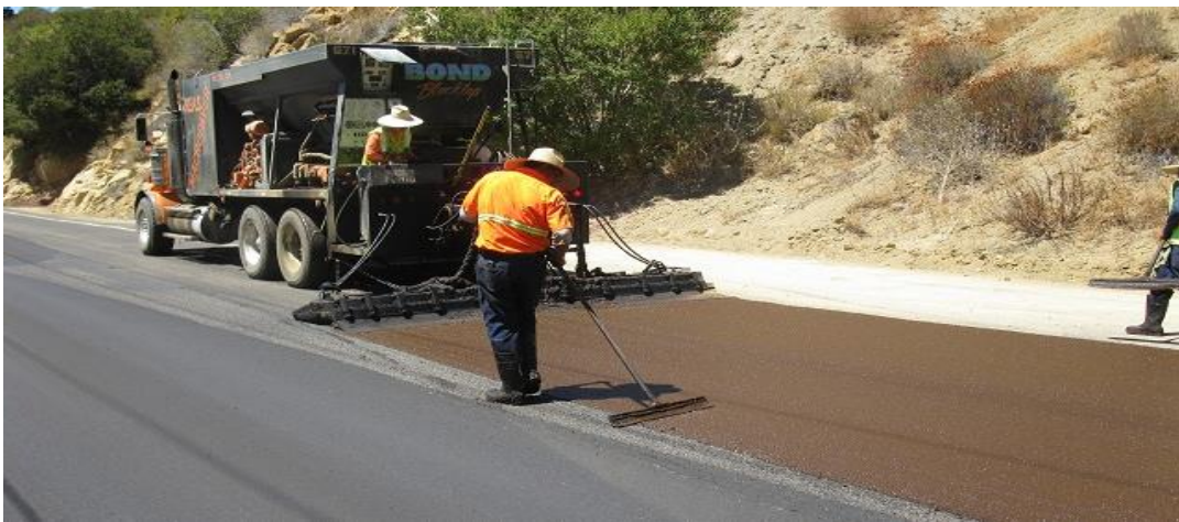
Figure 8.28 Photo Showing Micro-Surfacing
