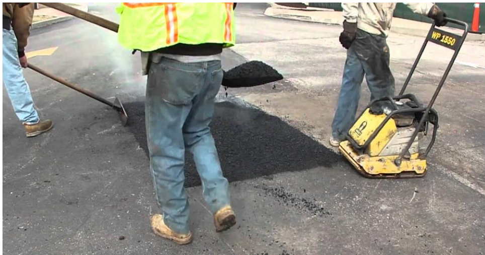
Figure 8.49 Photo of Manual Skin Patching
