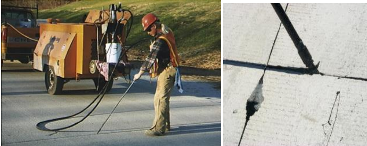
Figure 10.6 Photos of Concrete Joint Resealing
