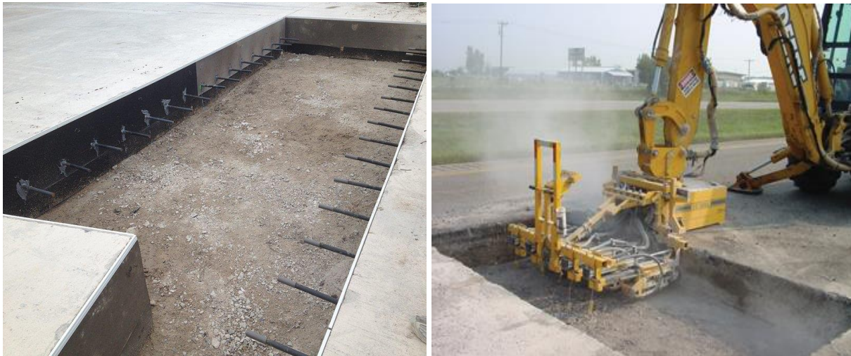
Figure 10.8 Photos of Full Depth Concrete Repair
