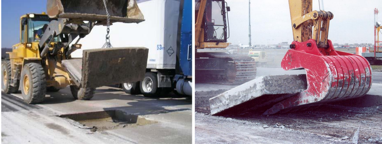
Figure 10.9 Photos of Concrete Slab Removal
