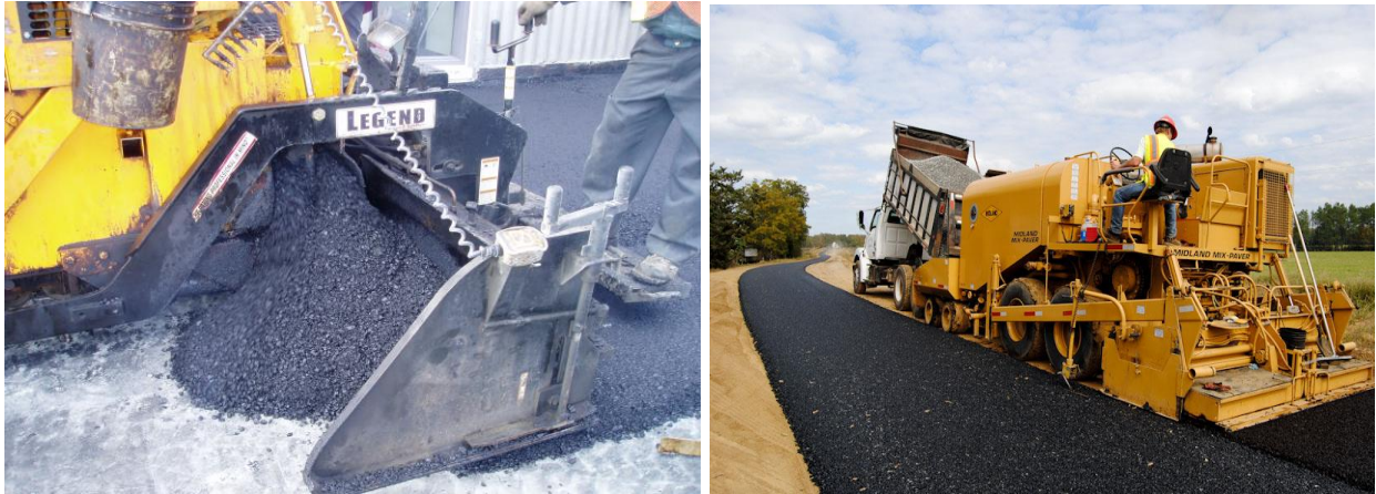
Figure 8.43 Photos of Cold Mix Paving
