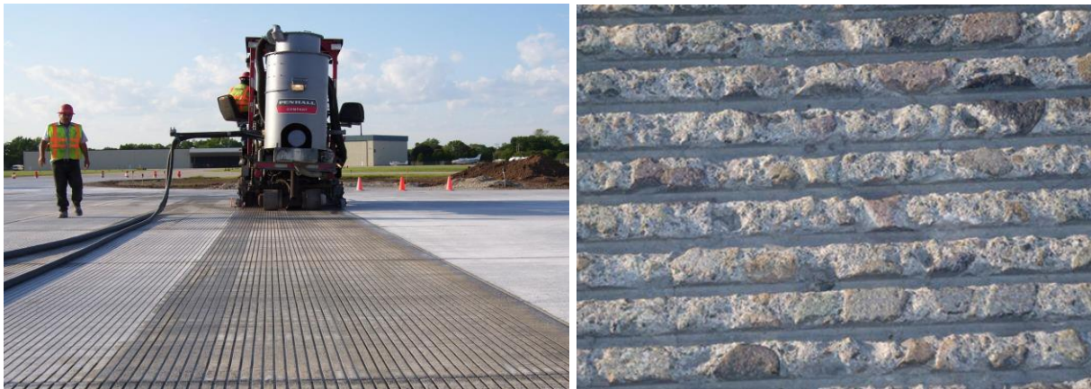
Figure 10.2 Photos of Diamond Grinding and Grooving
