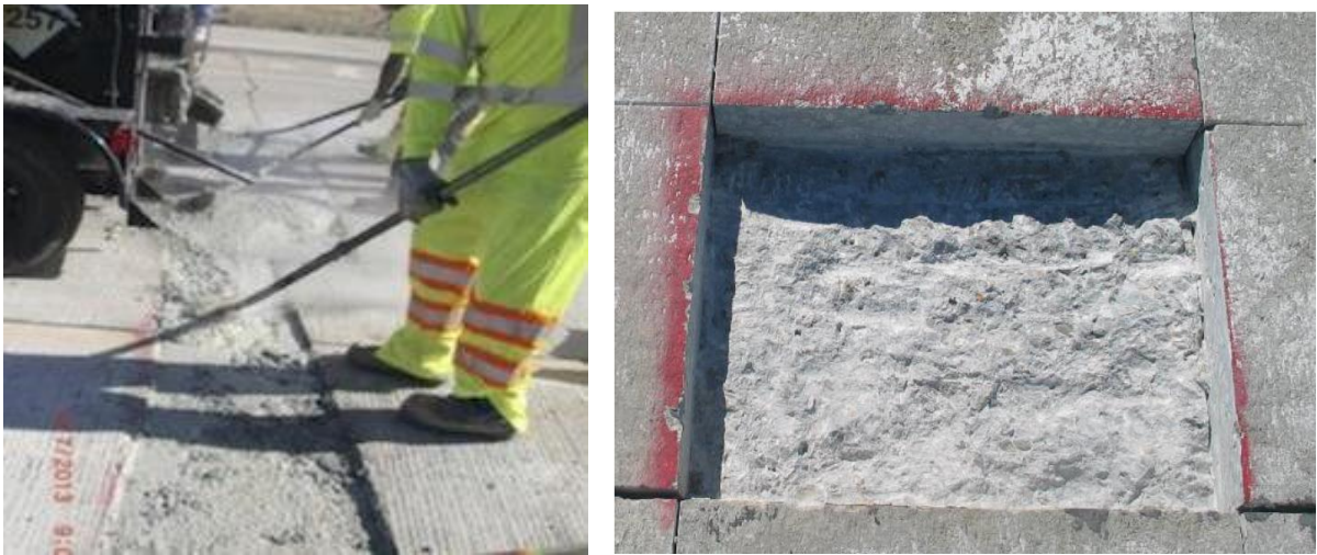
Figure 10.7 Photos of Partial Depth Concrete Repair
