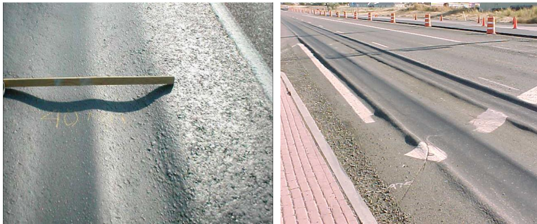
Figure 8.5 Photos of Rutting
