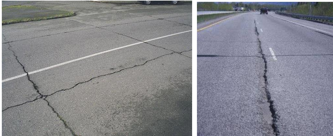
Figure 8.4 Photos of Longitudinal and Transverse Cracking
