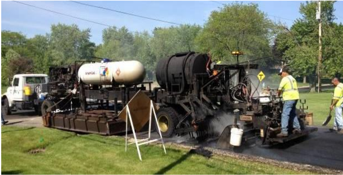
Figure 8.14 Photo of Heating Scarifying Equipment (Initial Operation)
