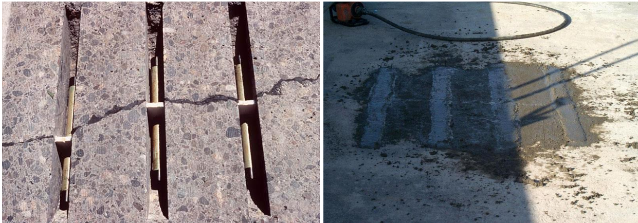
Figure 10.18 Photos of Slot Stitching
