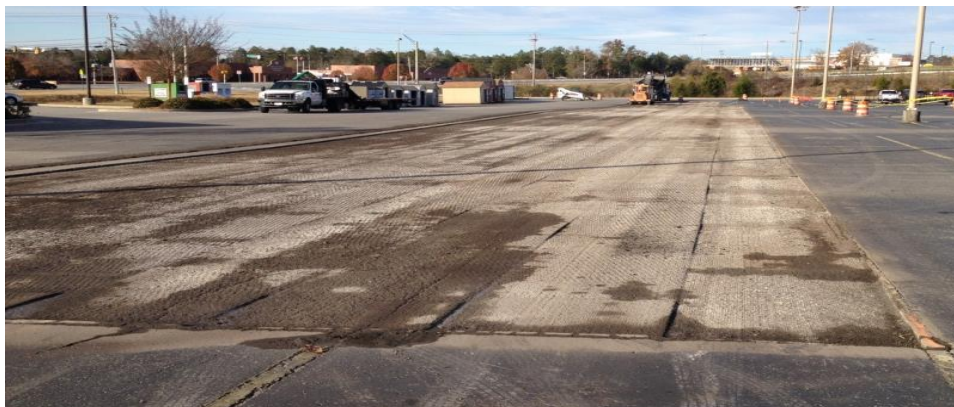
Figure 8.7 Photo of Milling of Old Asphalt
