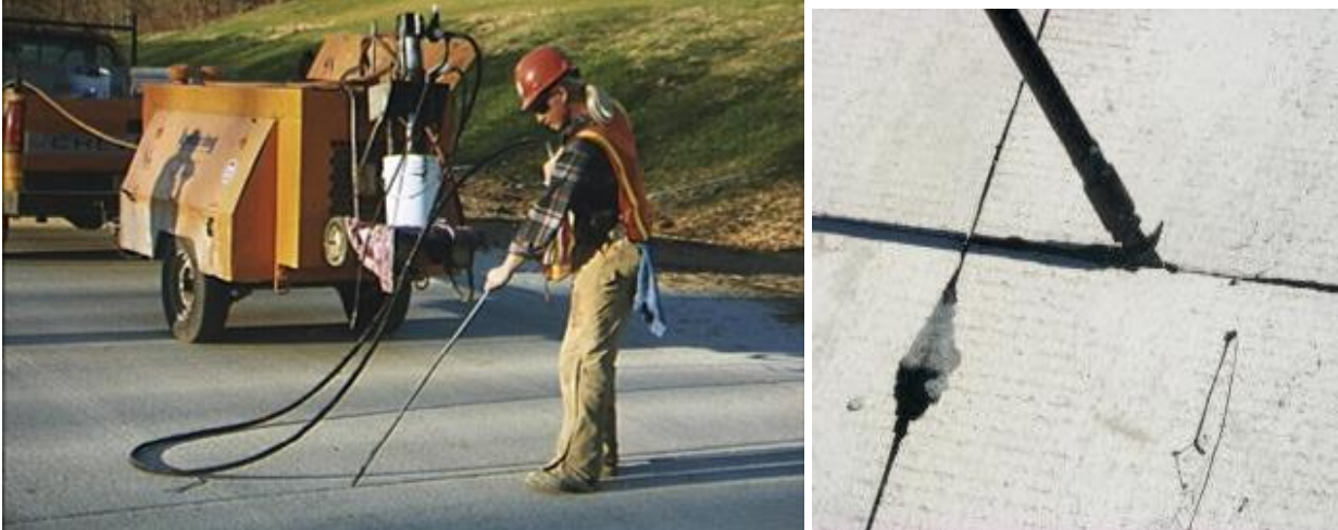
Figure 10.6 Photos of Concrete Joint Resealing
