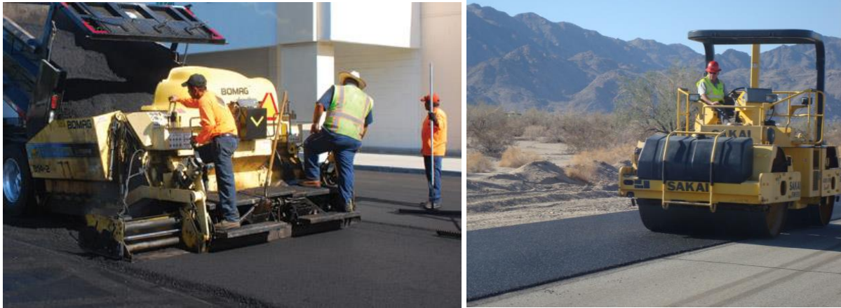
Figure 8.27 Photos of Typical HMA Overlay Equipment (Truck with Spreader and Roller)
