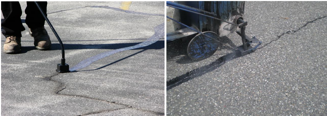
Figure 8.42 Photos Showing Crack Sealing
