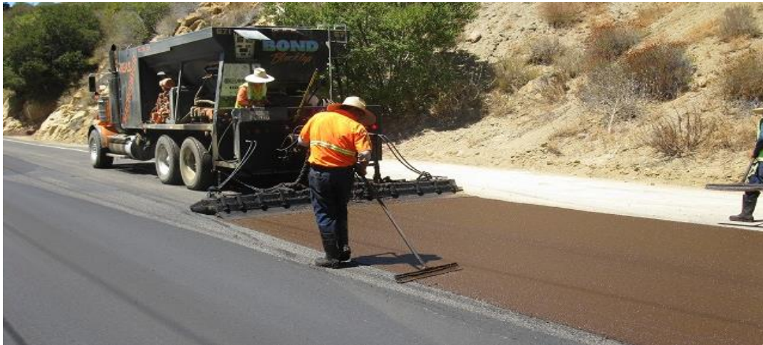
Figure 8.28 Photo Showing Micro-Surfacing
