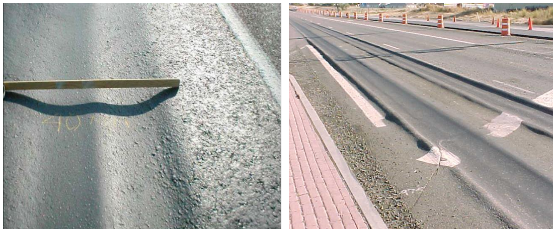
Figure 8.5 Photos of Rutting
