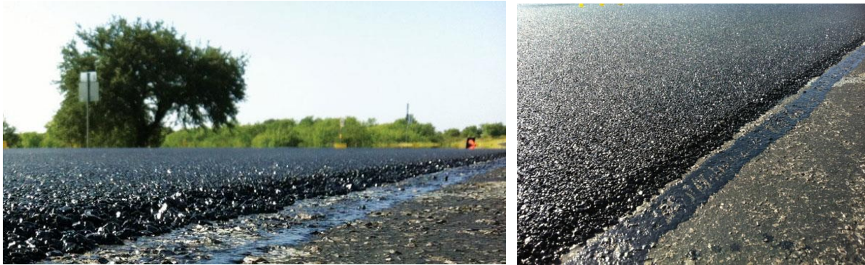
Figure 8.24 Conventional Hot Mix Asphalt (HMA) Layer
