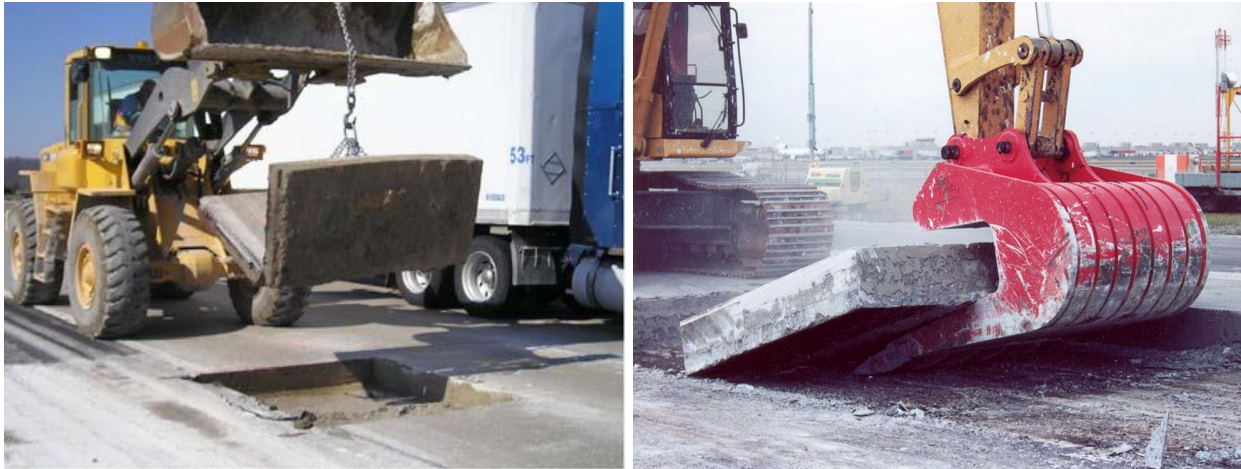
Figure 10.9 Photos of Concrete Slab Removal
