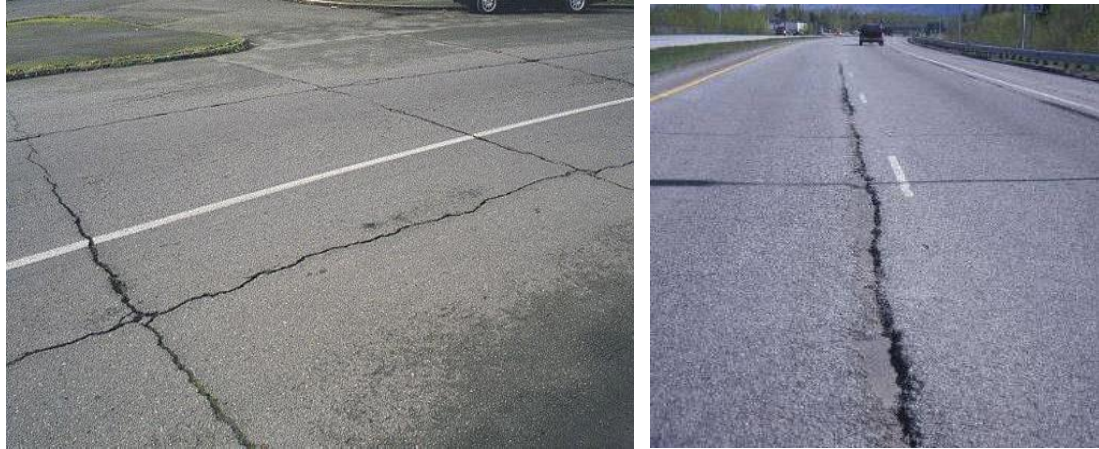
Figure 8.4 Photos of Longitudinal and Transverse Cracking
