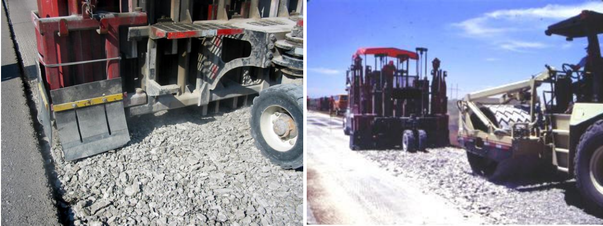
Figure 8.35 Photos of the Rubbilization Initial Operation
