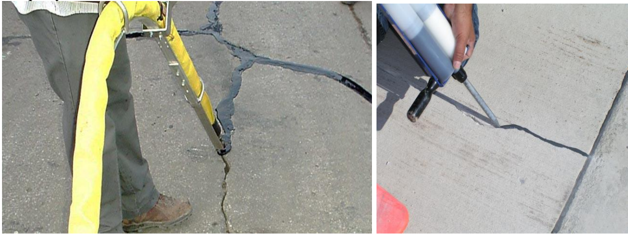
Figure 10.5 Photos of Crack Sealing
