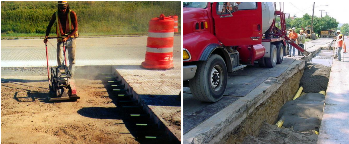
Figure 10.10 Photos of Compaction of Subbase and Flowfill Placement
