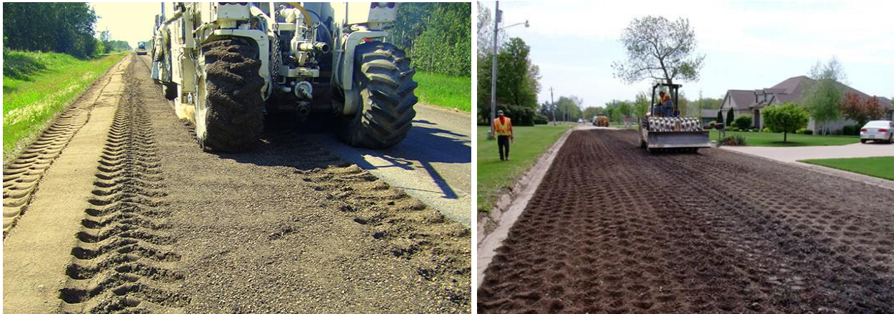
Figure 5.9 Photos of Full Depth Asphalt Reclaimed Base
