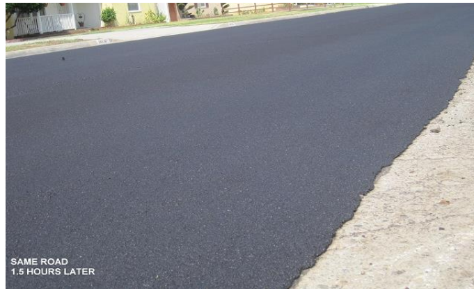
Figure 8.41 Photo Showing a Slurry Seal 1.5 Hours After Placement
