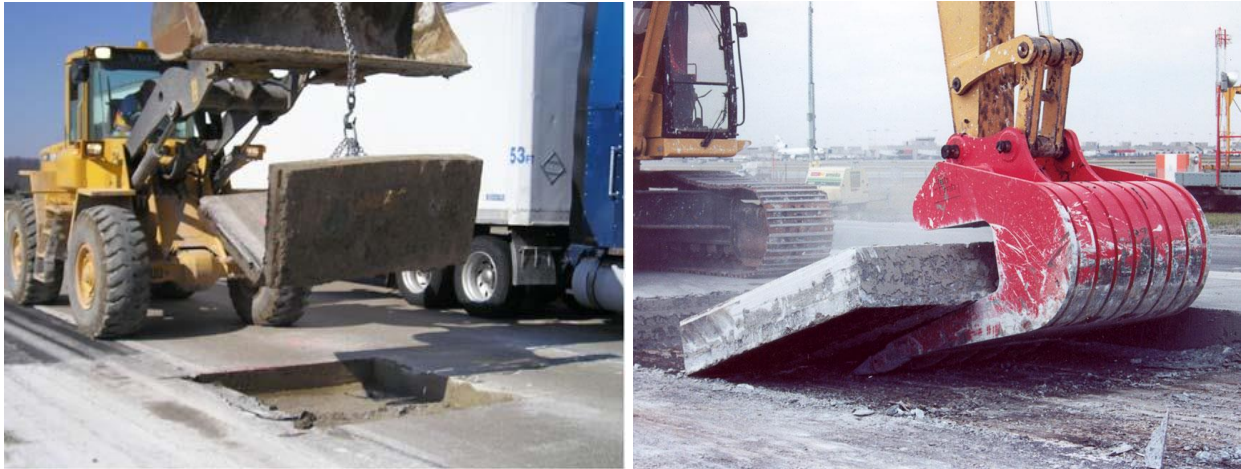
Figure 10.9 Photos of Concrete Slab Removal
