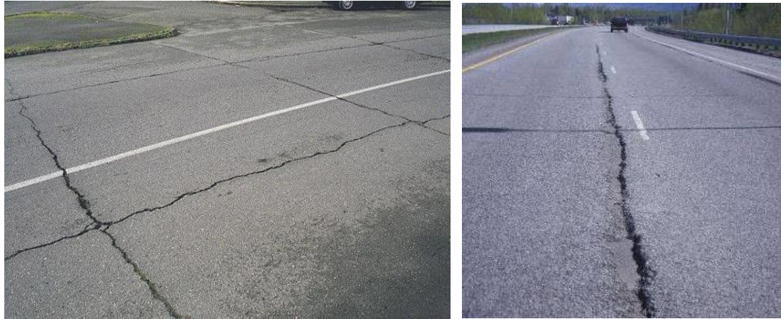
Figure 8.4 Photos of Longitudinal and Transverse Cracking
