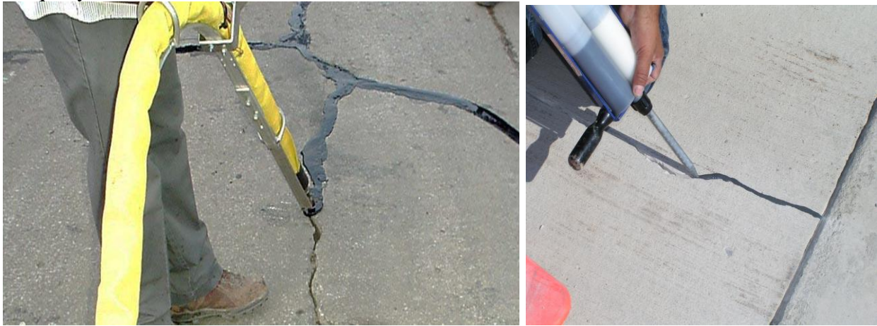
Figure 10.5 Photos of Crack Sealing
