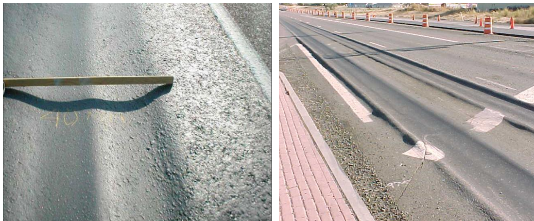
Figure 8.5 Photos of Rutting
