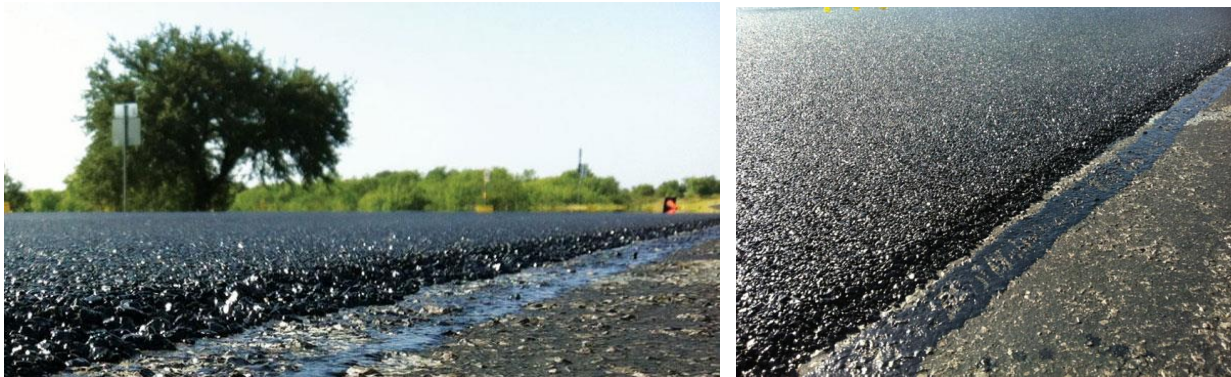
Figure 8.24 Conventional Hot Mix Asphalt (HMA) Layer
