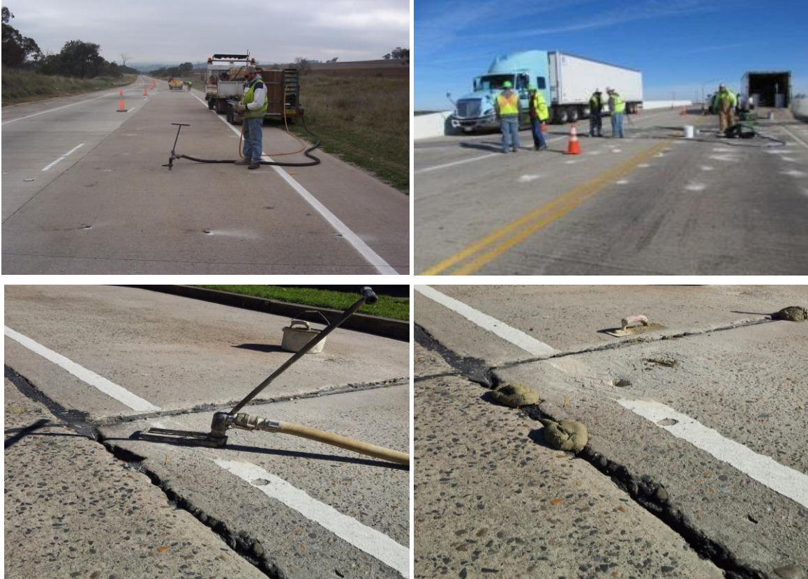
Figure 10.22 Photos of Slabjacking
