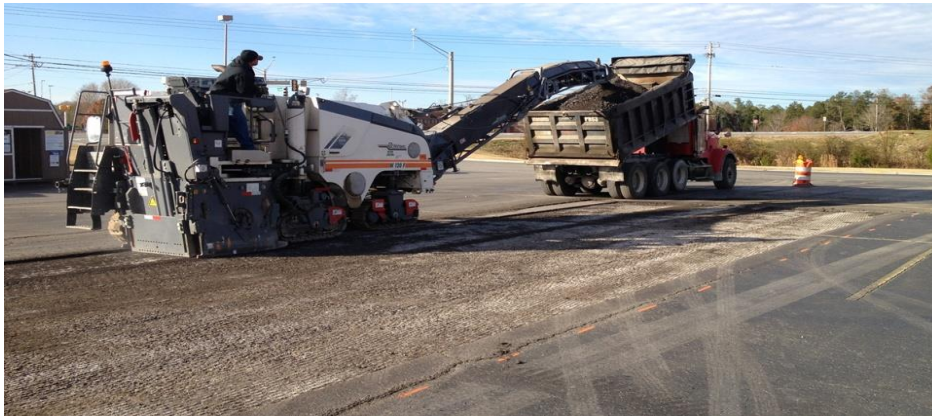
Figure 8.7 Photo of Milling of Old Asphalt
