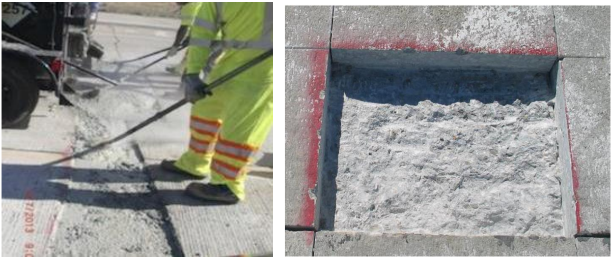
Figure 10.7 Photos of Partial Depth Concrete Repair
