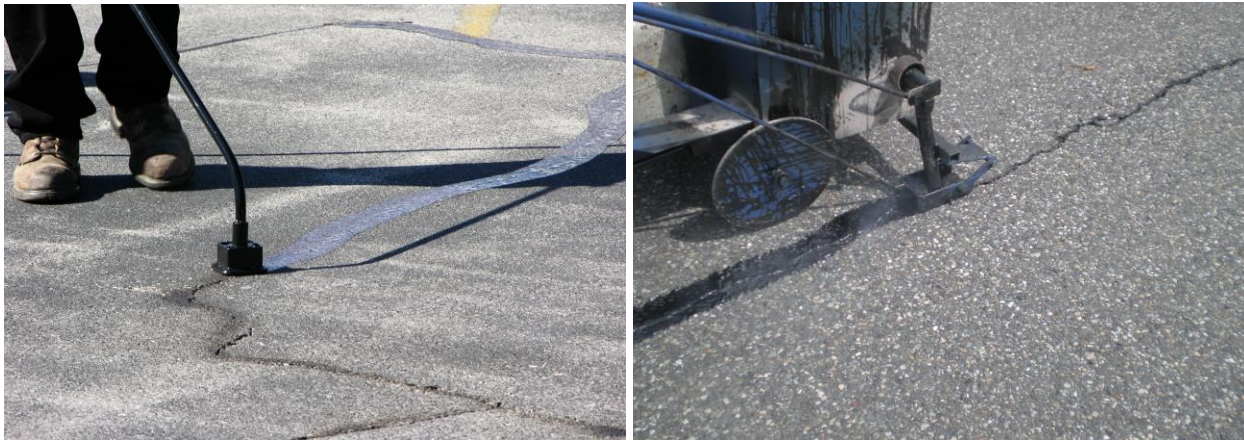
Figure 8.42 Photos Showing Crack Sealing
