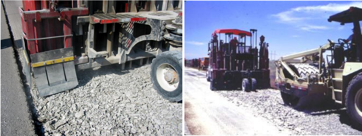
Figure 8.35 Photos of the Rubbilization Initial Operation
