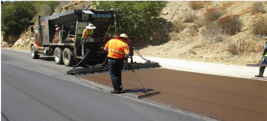
Figure 8.28 Photo Showing Micro-Surfacing
