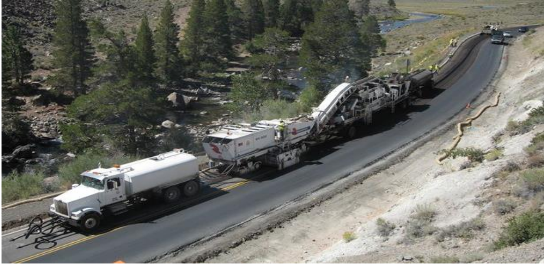
Figure 8.46 Photo Showing A Cold In-Place Recycling Operation
