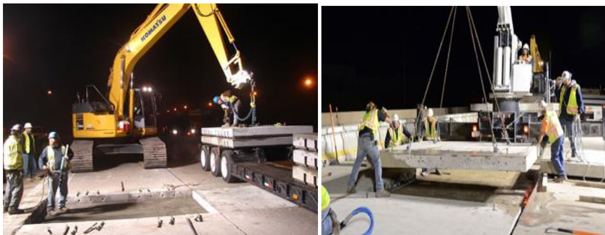
Figure 10.13 Photos of Precast Concrete Panel Repair
