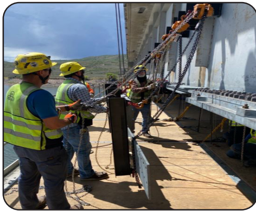
Image 5. Repair Plate Installation
