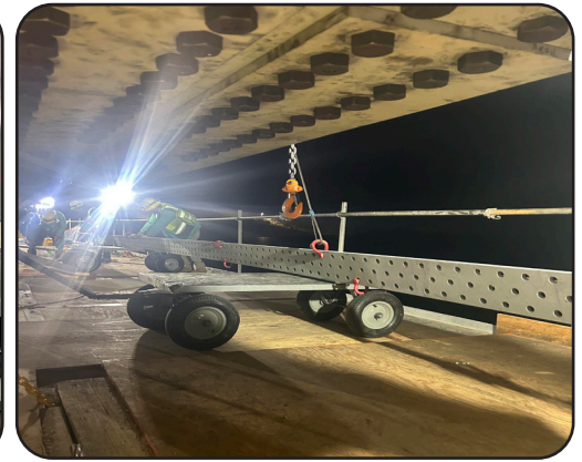
Image 7. Crack Arrest Plate Positioning
