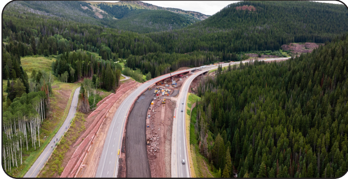
Image 24. New Completed Bridge of I-70 WB over Polk Creek
