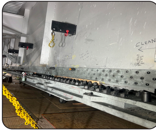
Image 6. Crack Arrest Plate Hung
