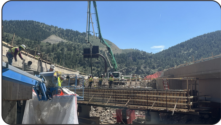
Image 26. Placing Girders for the Temporary Floyd Hill Bridge
