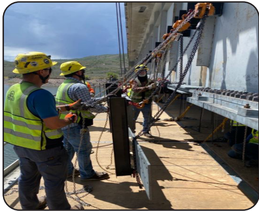
Image 5. Repair Plate Installation
