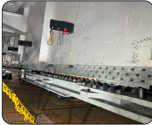
Image 6. Crack Arrest Plate Hung
