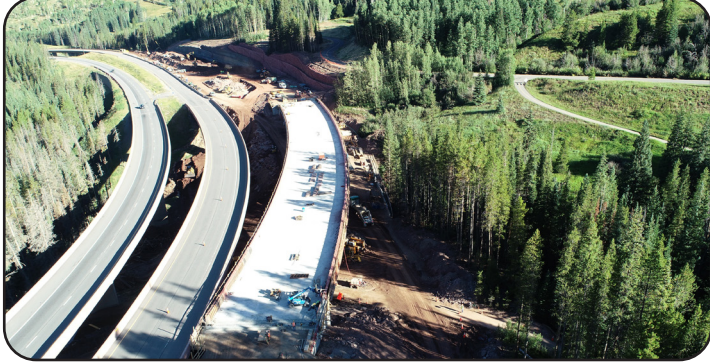
Image 27. New Bridge Deck of I-70 WB over Polk Creek
