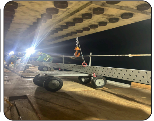
Image 7. Crack Arrest Plate Positioning
