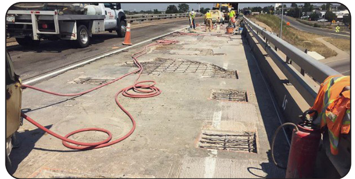
Image 28. Emergency Repairs on I-270
