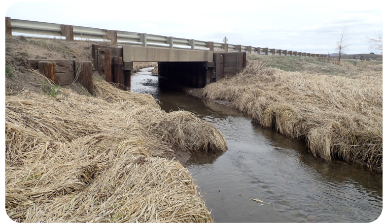
Image 9. US 40 ML over Shelton Ditch (C-08-A_Minor)
