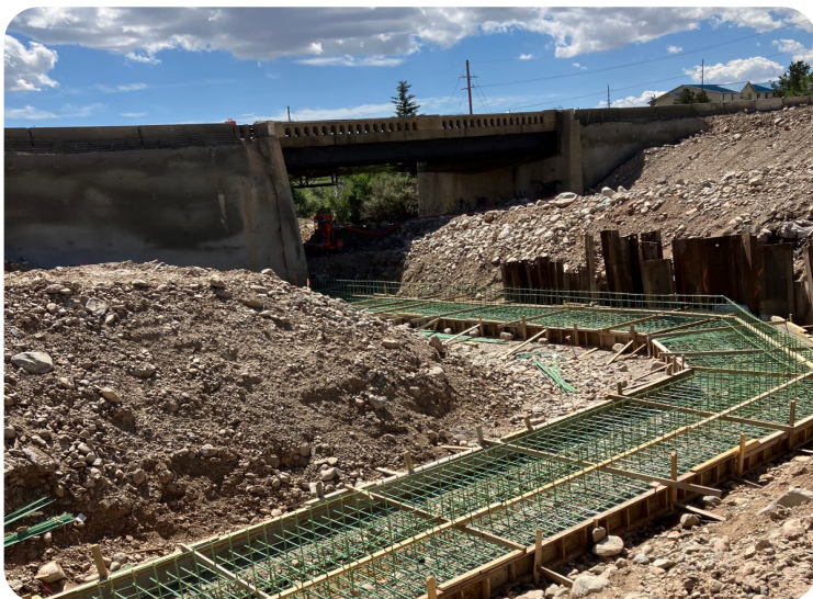
Image 29. Retaining Wall Footer Adjacent to the Bridge
