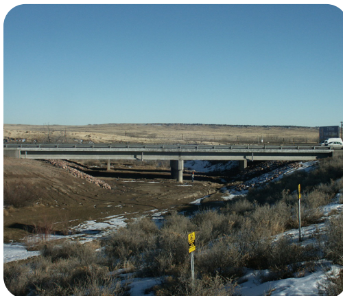
Image 21. US 50 WBND over Six Mile Creek
