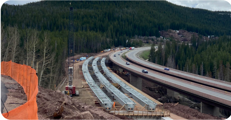
Image 23 & 24. New bridge girders for the future westbound bridge at I-70 WB over Polk Creek (F-12-AT)
