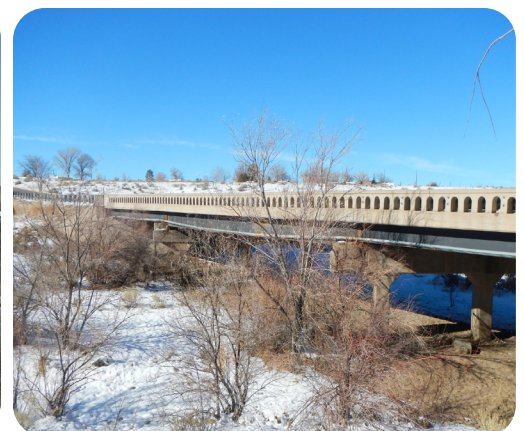
Image 22. I-25 Bus Rt over Bear Creek
