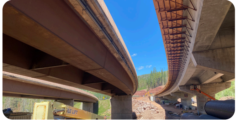
Image 23 & 24. New bridge girders for the future westbound bridge at I-70 WB over Polk Creek (F-12-AT)
