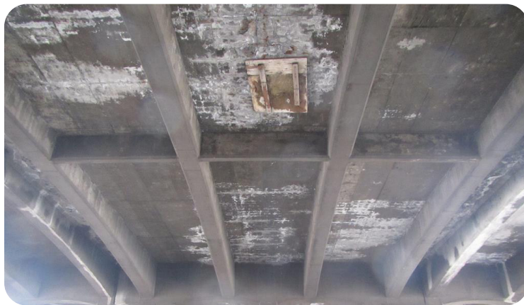
Image 9. Deck Patch on US 6 over SH 121 (F-16-O)
