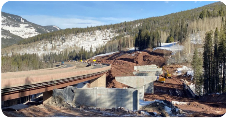
Image 20 & 21. New Bridge Piers and Abutments for the Future Westbound Bridge at I-70 WB over Polk Creek (F-12-AT)
