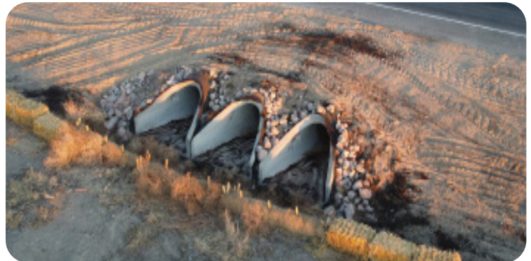
Image 24. Construction at US 350 over Draw (M-22-Y)
