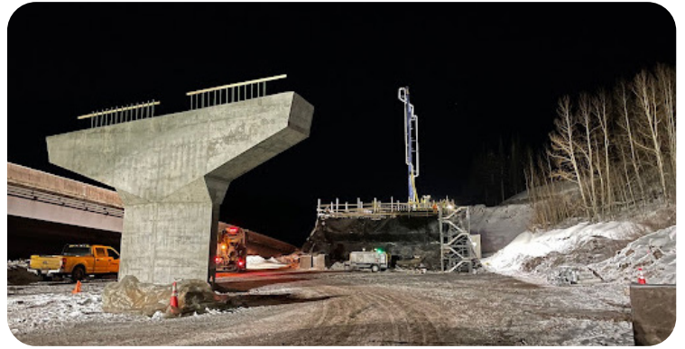
Image 20 & 21. New Bridge Piers and Abutments for the Future Westbound Bridge at I-70 WB over Polk Creek (F-12-AT)
