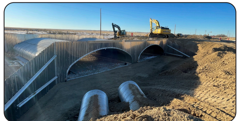
Image 20. Construction on US 350 over Draw
