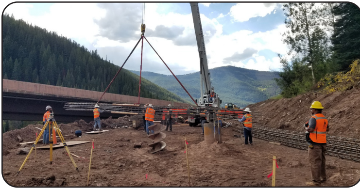
Image 16 & 17. Drilled Shafts and Setting Rebar Cages for Pier 2 at I-70 WB over Polk Creek (F-12-AT)
