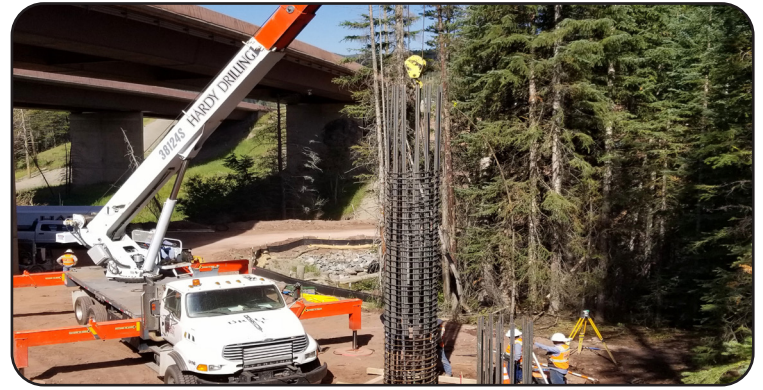
Image 16 & 17. Drilled Shafts and Setting Rebar Cages for Pier 2 at I-70 WB over Polk Creek (F-12-AT)
